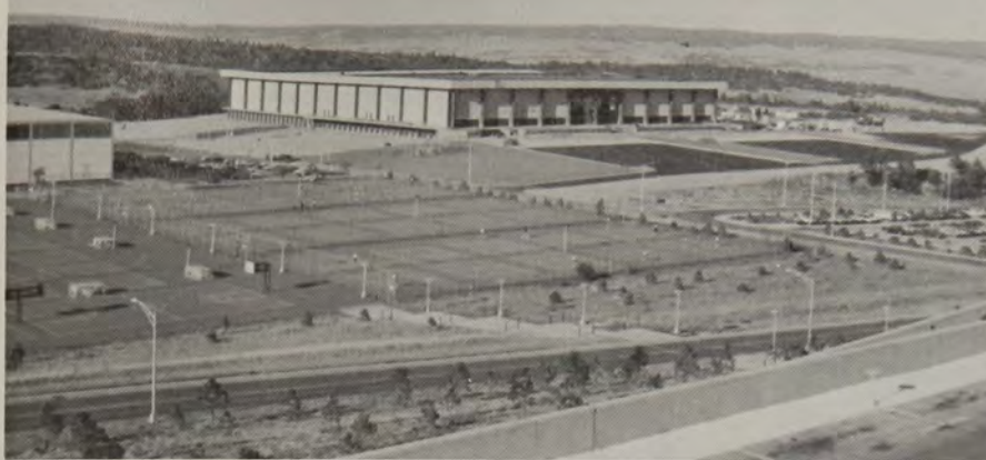
The new fieldhouse nears completion.
