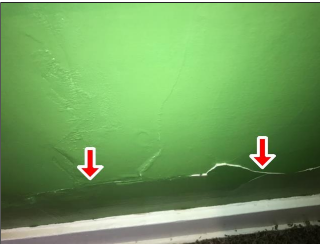
9.2 Wall Cracking
