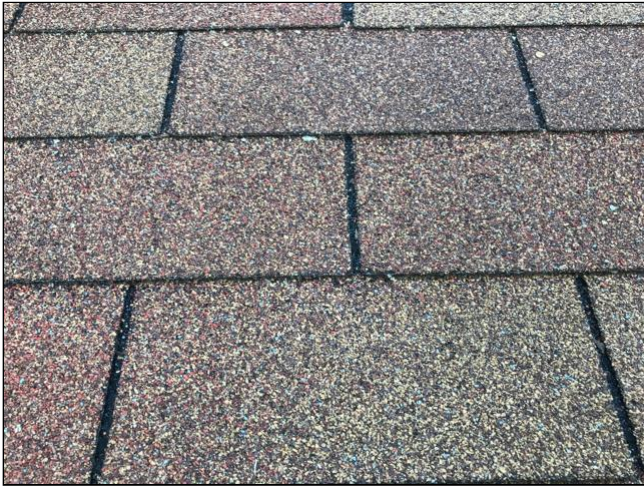
2.2 Asphalt/Fiberglass Shingles
