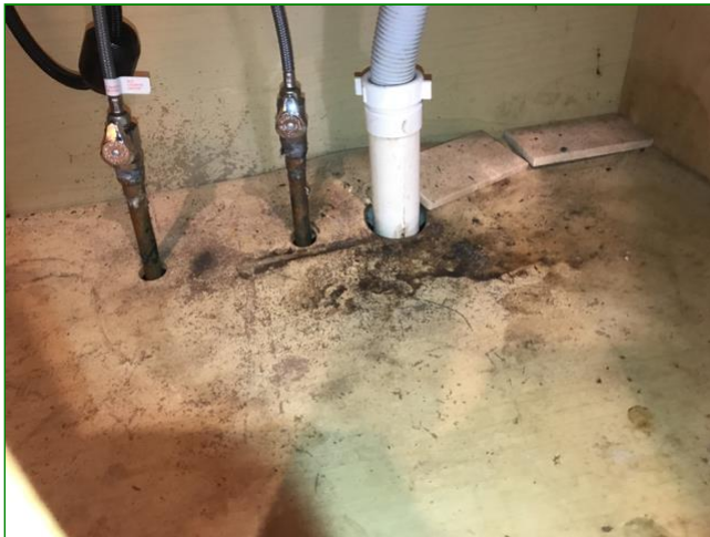
Item 8 - Deteriorated Cabinet Floor
