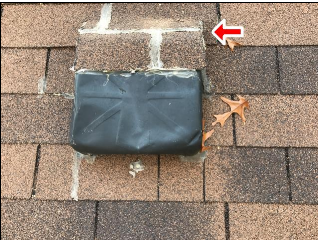
2.6 Improperly Installed Roof Vent
