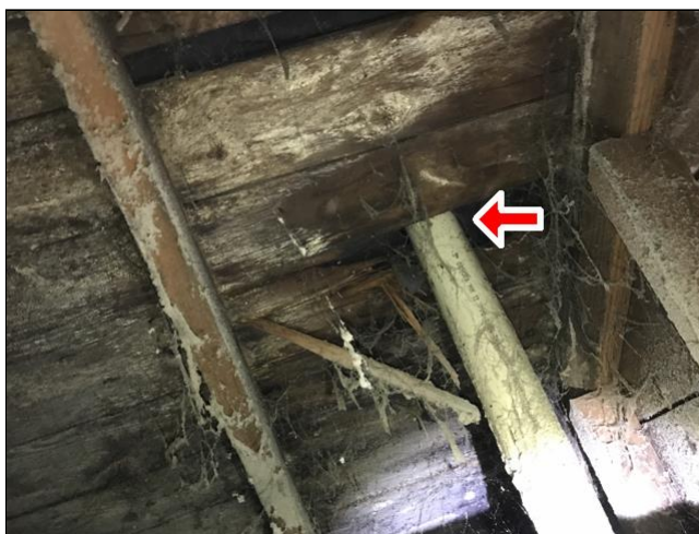
4.2 Pipe Vent Penetration
