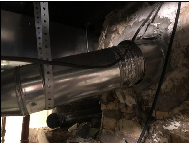
14.7 Furnace Exhaust Stack
