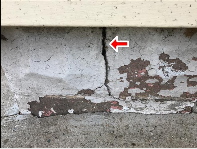
1.12 Foundation Crack
