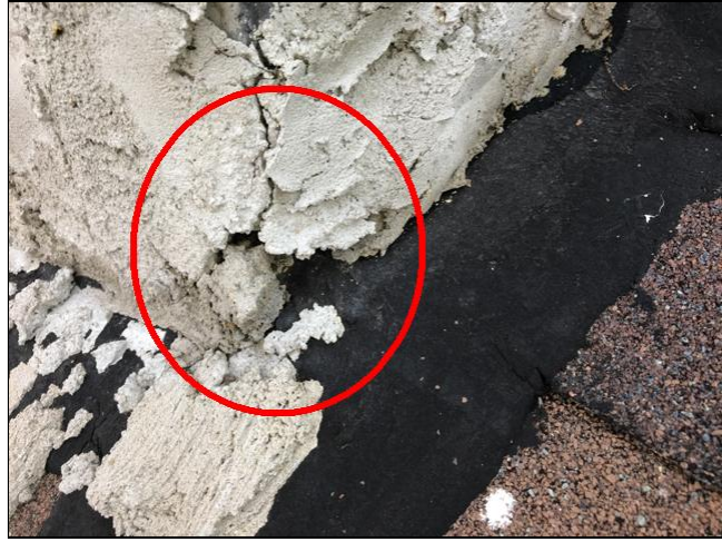
2.4 Cracking Stucco
