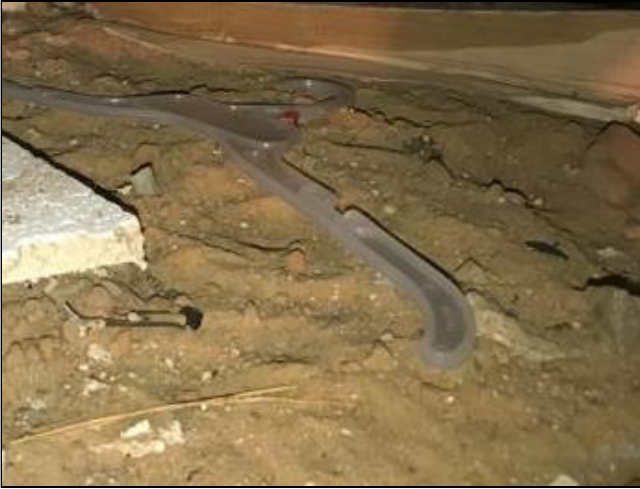
11.6 Missing Vapor Barrier
