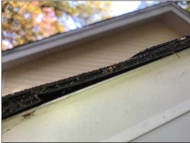
2.2 Single Layer of Shingles
