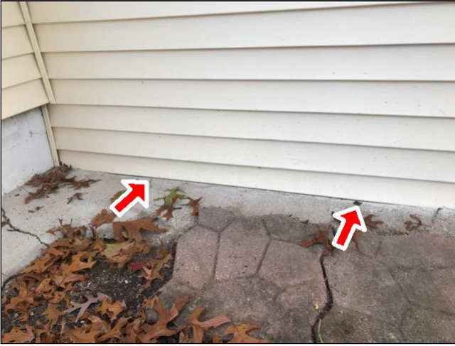
1.4 Siding at Ground Level
