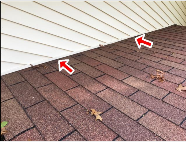
2.5 Roof Flashing
