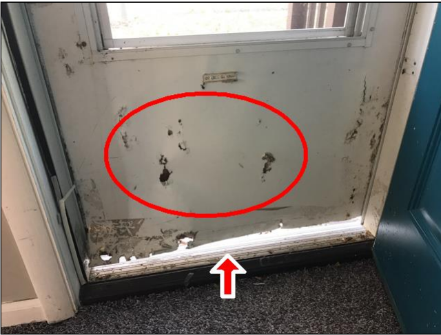
5.3 Damaged Storm Door
