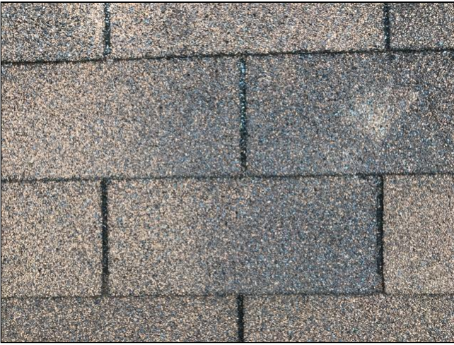
2.2 Asphalt/Fiberglass Shingles
