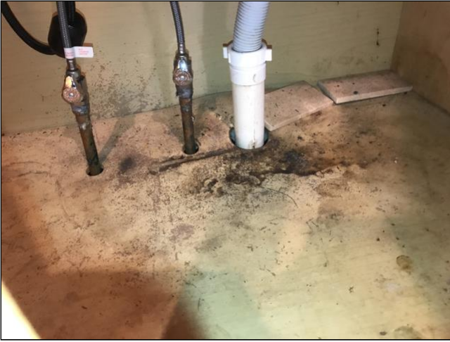
6.8 Deteriorated Cabinet Floor
