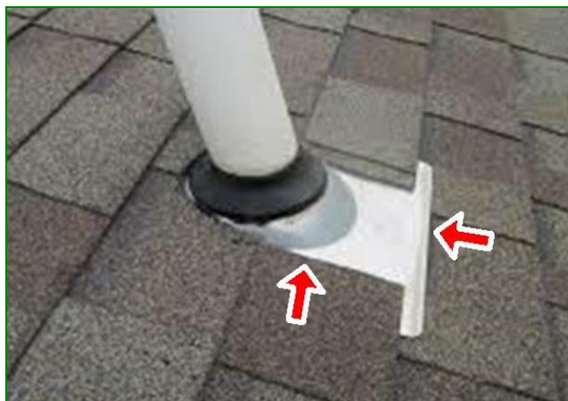
Item 3 - Example: Properly Installed Pipe Vent Boot
