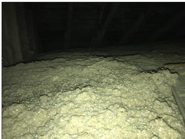
4.3 Cellulose Insulation
