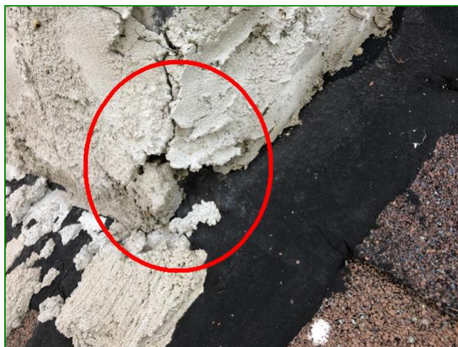
Item 4 - Cracking Stucco
