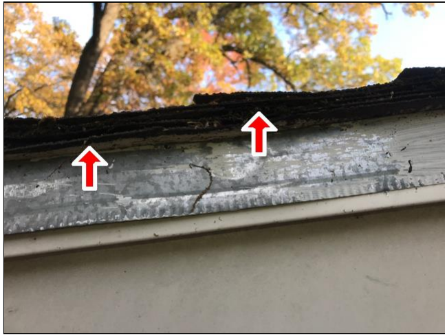
2.2 Two Layers of Shingles
