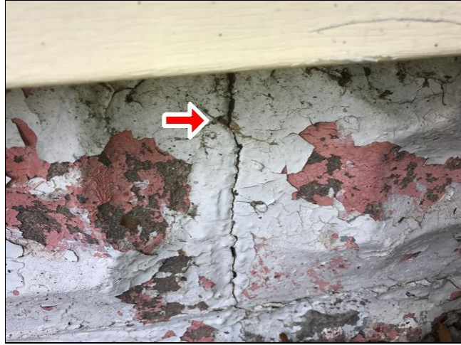
1.12 Foundation Crack
