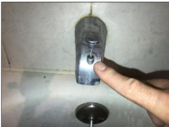
10.10 Stuck Water Flow Diverter
