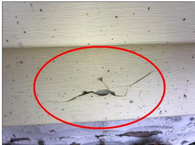
1.4 Cracked Siding
