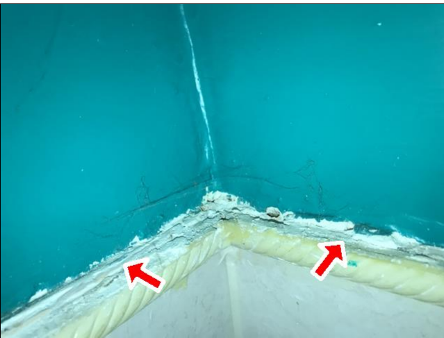
10.2 Deteriorating Caulk
