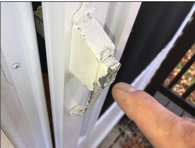
6.5 Damaged Exterior Handle
