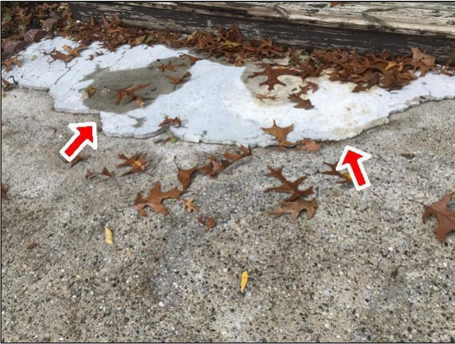
1.1 Poor Surface Patch
