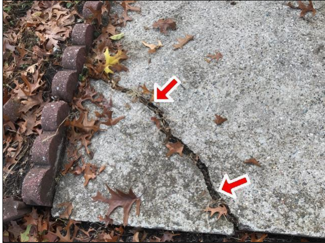
1.1 Cracked & Sunken Corner
