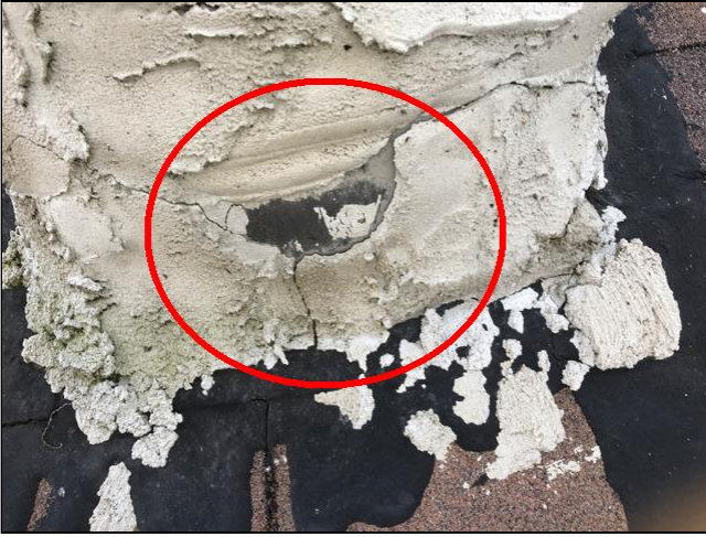
2.4 Deteriorating Stucco
