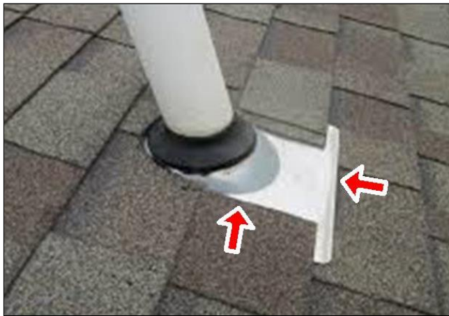
2.3 Example: Properly Installed Pipe Vent Boot
