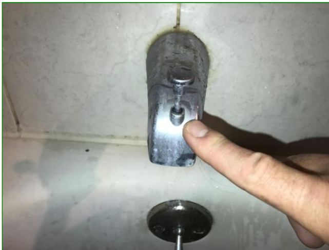
Item 12 - Stuck Water Flow Diverter
