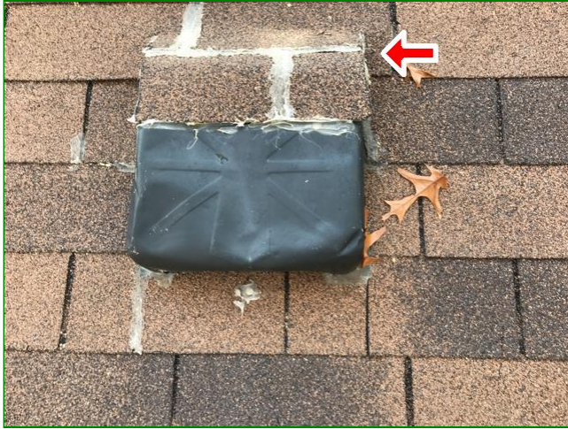
Item 5 - Improperly Installed Roof Vent
