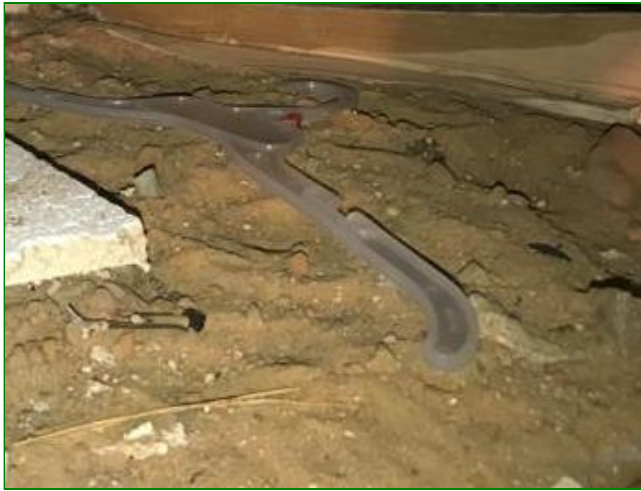
Item 13 - Missing Vapor Barrier
