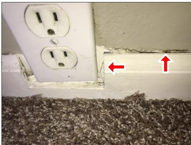
5.2 Crudely Installed Trim & Wall Cracking
