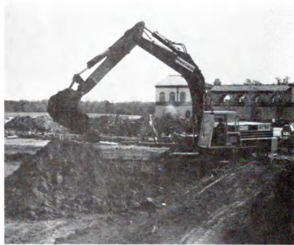
Back-hoe equipment was utilized for the trenching operations necessary to lay and connect main sewer lines. The present Unity Inn is shown in the background.
