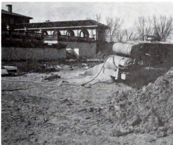
A rock ledge underlying the parking lot required large air compressor units to power the pneumatic jackhammers necessary to complete the trenching operation.
