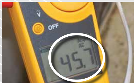
Amp measurement with 5-2-1 ® Compressor Saver ®
