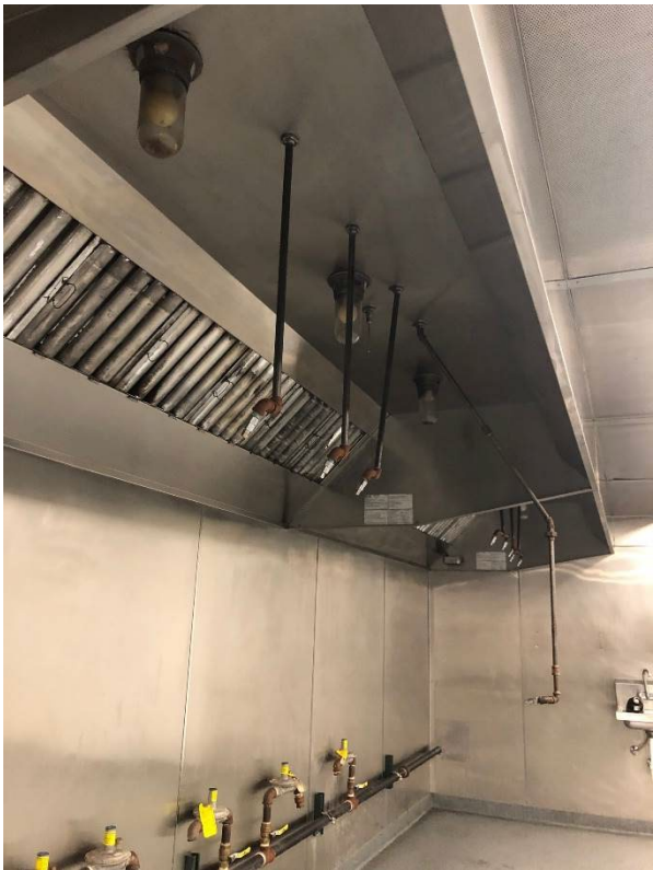
Exhaust Hood with Fire Protection
