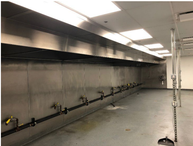
Exhaust Hood with Fire Protection
