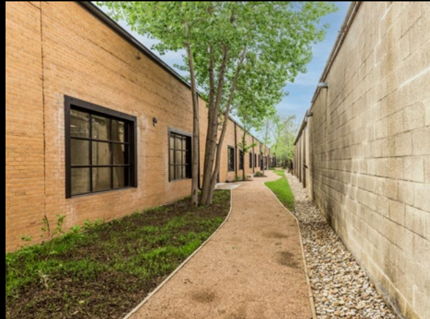
The Rail Spur
