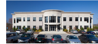
HENRY COUNTY MEDICAL OFFICE BUILDING
