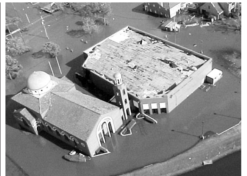
Holy Trinity Cathedral suffered damage during Hurricane Katrina.
