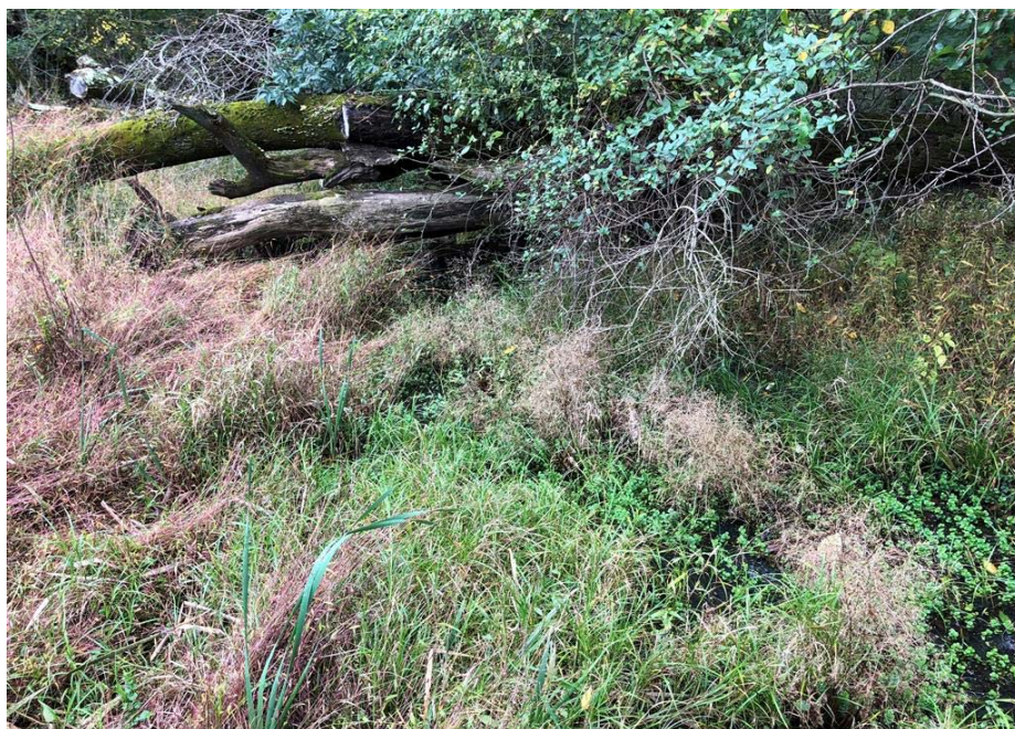
Picture 5 – Standing water at toe of slope of the polishing pond.
