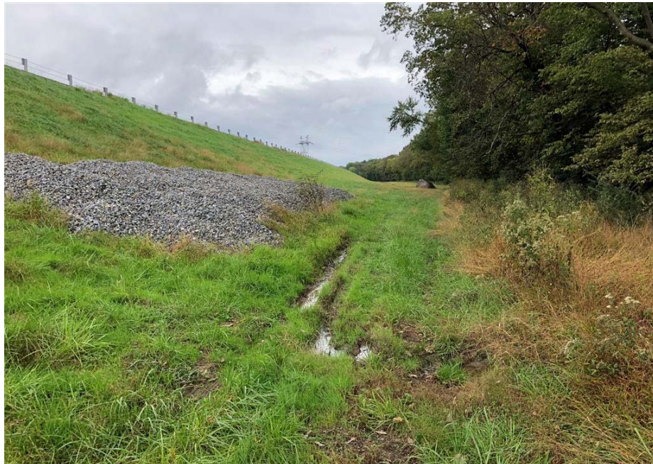
Picture 7 –Weighted filter blanket at the SE corner.
