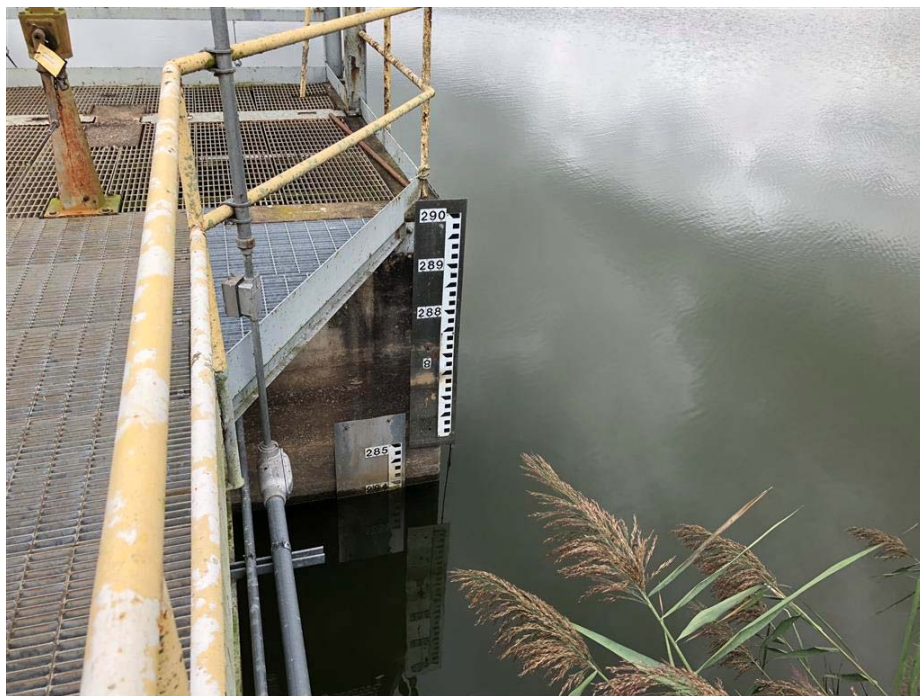
Picture 14 – Staff gage on side of structure.
