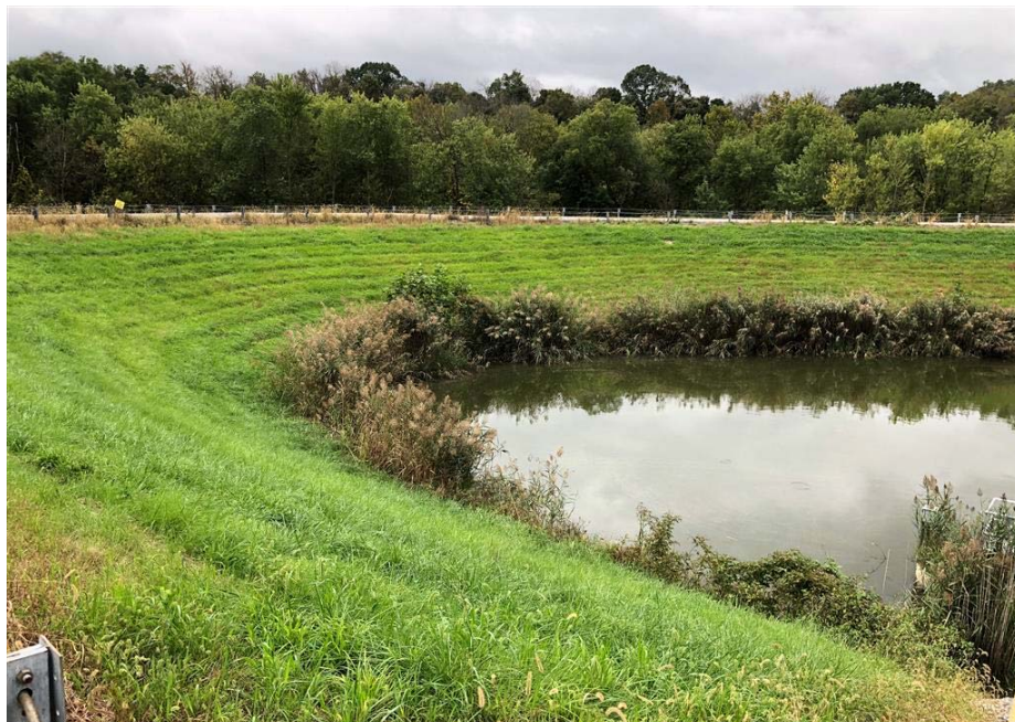
Picture 11 – Vegetation should be cut and removed from the water's edge around the polishing pond.
