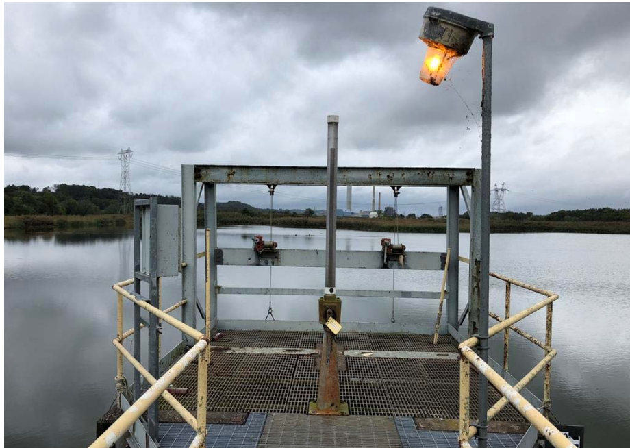
Picture 13 – Gate open and locked.
