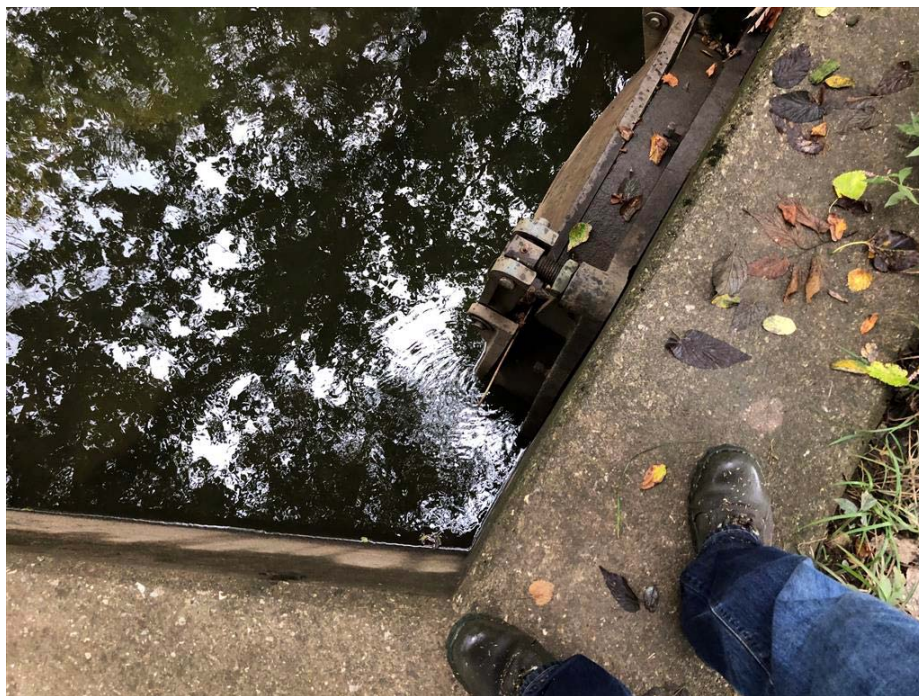
Picture 6 –No issues observed at the discharge.
