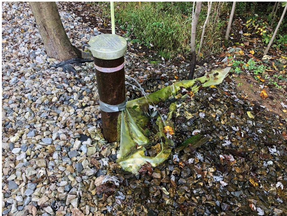
Picture 4 – Well in artesian condition. The flowing water showed no signs of turbidity.
