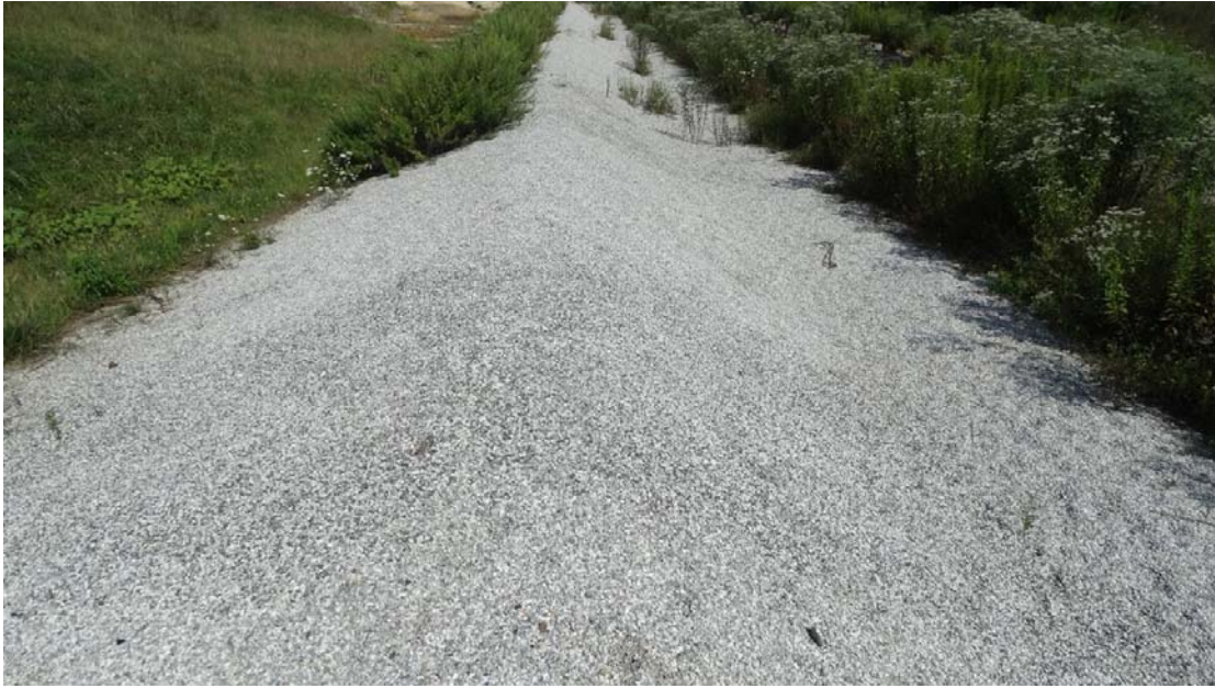
Picture 11 – Berm between Cell 1 and future Cell 2. A geo-membrane rain flap liner has been installed separating the two cells. The liner was exposed in a few areas.
