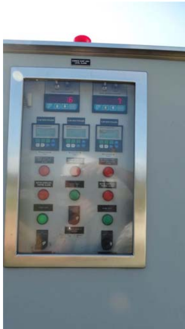
Picture 15 – Control board showing the pumps with runtime, flow meters, and depth of water in the leachate collection zone and the leak detections zone.
