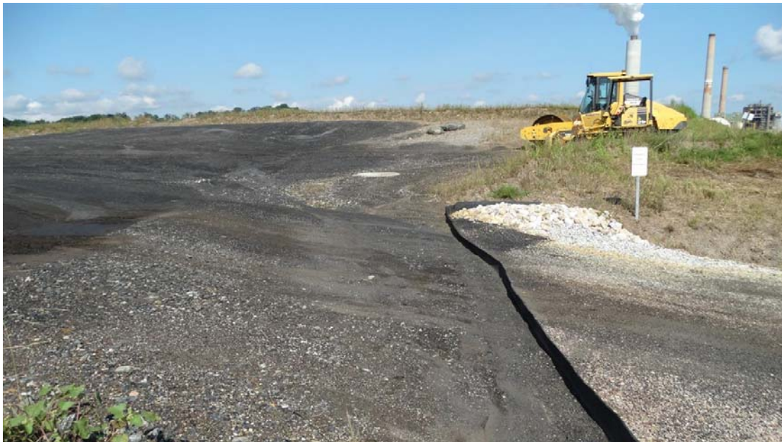
Picture 3 – Erosion scar in the recently regraded slope above the entrance road.
