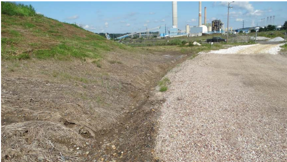
Picture 1 – New sand and rock filter around the sump area to reduce the sediment in the sump area.
