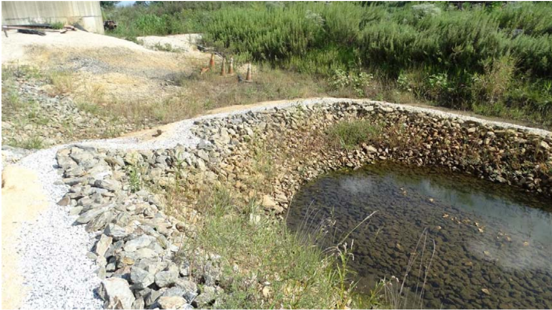
Picture 1 – New sand and rock filter around the sump area to reduce the sediment in the sump area.
