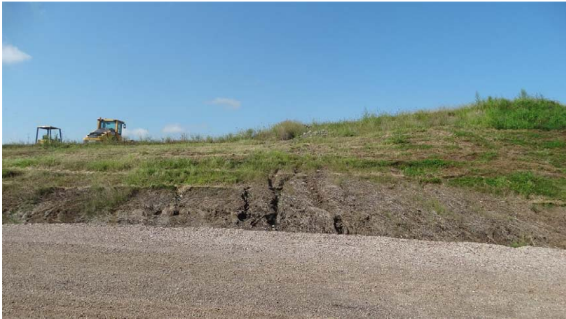
Picture 3 – Erosion scar in the recently regraded slope above the entrance road.
