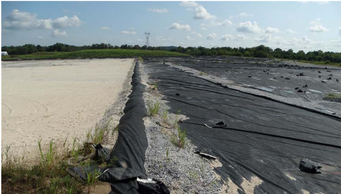
Picture 9 – Recently relocated separation berm between inactive and active portions of the landfill.
