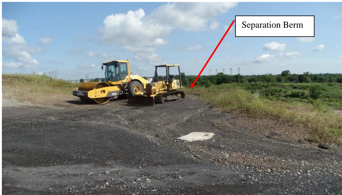
Picture 5 – Berm behind the equipment is less than 2' high.
