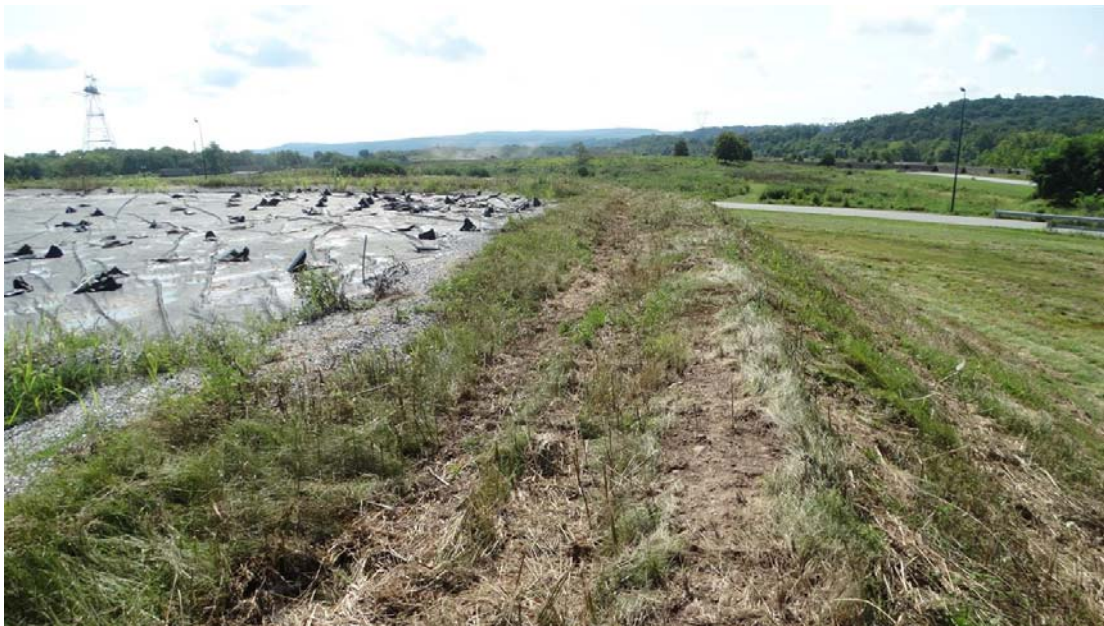
Picture 9 – Recently relocated separation berm between inactive and active portions of the landfill.
