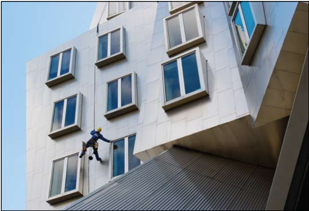
On Sept. 23, workers applied devices for reducing the buildup of snow and ice to the flat tops of windows that jut out from the Stata Center. MIT is currently suing architect Frank Gehry over the design of the building, after experiencing “persistent leaks” and “poor drainage.”
