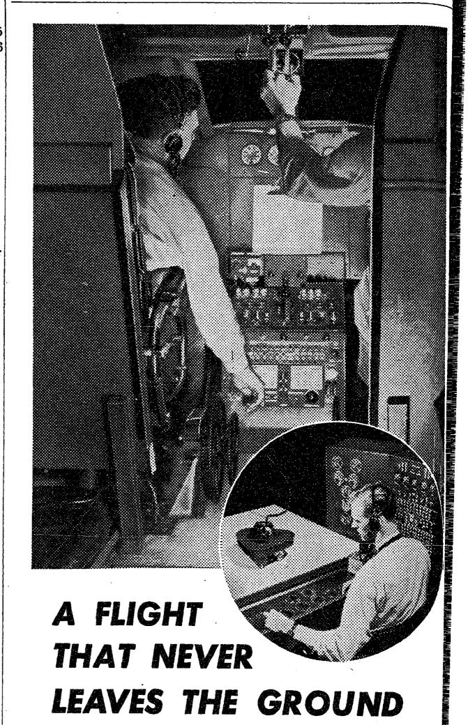
A bomber crew needs training as a team. And now those hazards which are too dangerous for air-borne drill can be duplicated on the ground. This is made possible by an electronic flight trainer perfected by Bell Telephone Laboratories' scientists for the Navy.
