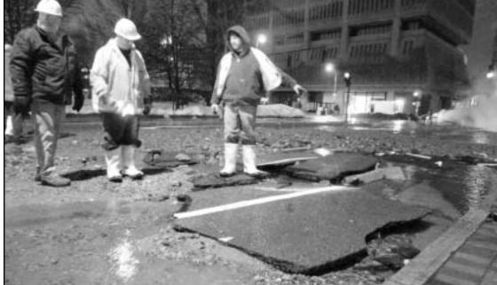
A Massachusetts Water Resources Authority employee points at a deep fissure in the asphalt near where a water main broke last night. The broken water main flooded Broadway with water and silt, and also disrupted water service to much of Cambridge and the MIT campus.
