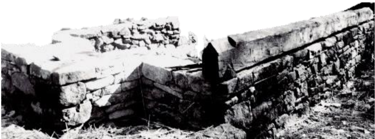
Figure 21. Stone foundation & V-shaped log notches
