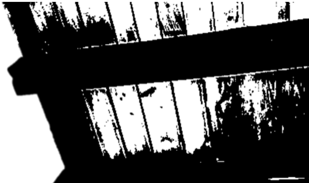
Figure 69. Ship-lapped ceiling
