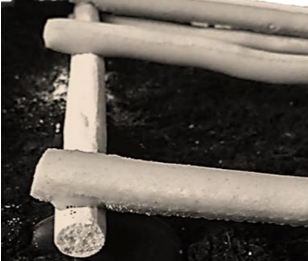
Figure 2. Round-shaped logs on a stone foundation
