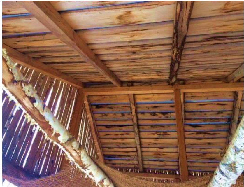
Figure 34. Roof boards for coverage
