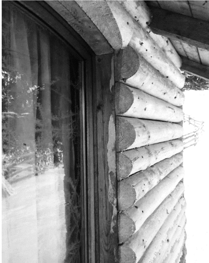
Figure 25. Window framing
