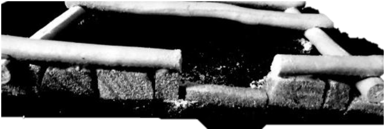
Figure 17. Stone foundation
