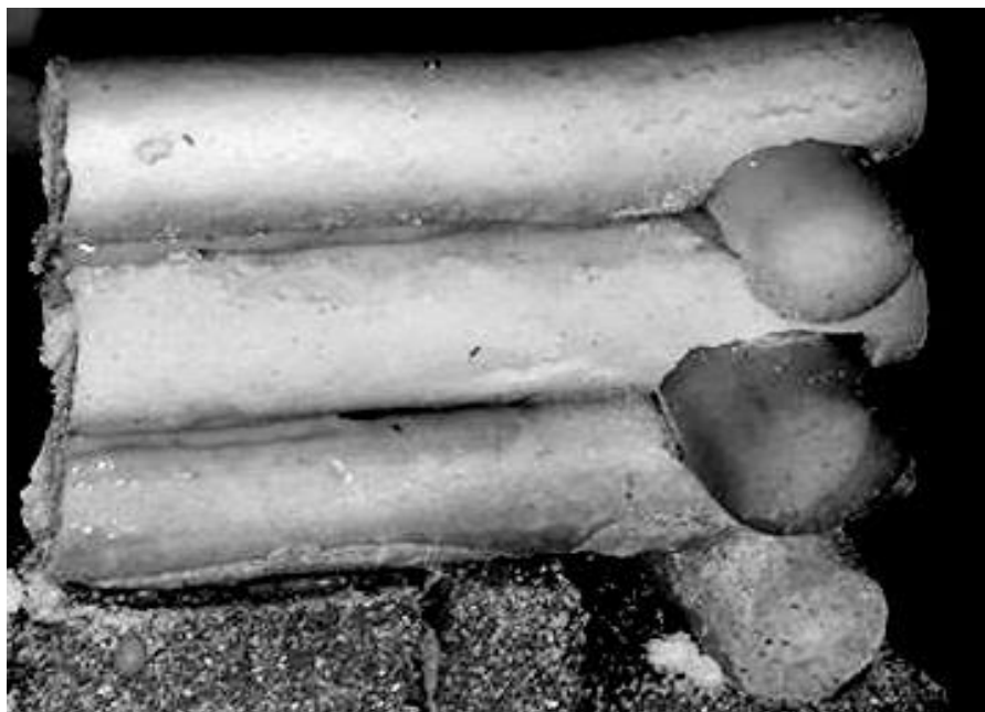
Figure 20. Log notching on round-shaped logs
