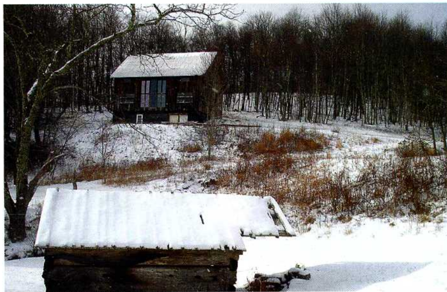
From palace to barn. The barn into which the royal flooring is being incorporated is a late 19th-century timber frame barn I bought on eBay; it was in the middle of a field near Quincy Ill., and was probably built as a kit in the Deep South (it's all Southern yellow pine heartwood), then shipped up the river. It was disassembled and arrived on the back of a giant flatbed truck six months later. I began re-erecting it on Thanksgiving in 2006.
