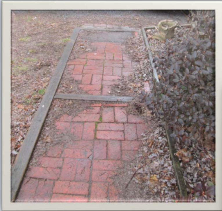
Sidewalk Repair Sullivan County
