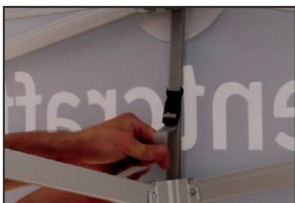
Pull the strap on the buckle to tighten the valance strap until the valance is taut. Repeat these two steps for the remaining three legs. **\*\*When taking the tent down, be sure to unbuckle these valance straps.\*\***
