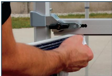
Unfold the half-wall and locate the top edge that is lined with white keder (a small plastic cylinder sewn into the top edge of the wall). Slide this keder into the track found along the bottom edge of the half-wall bar.
