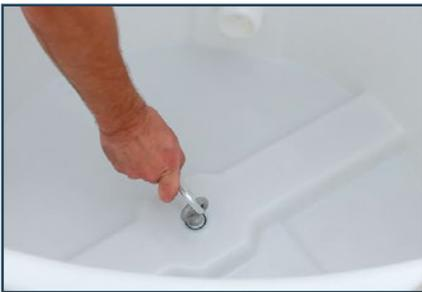
Connect the bottom carabiner on the outguy strap to the metal loop that is located on the bottom of the inside of the water barrel. Be sure that the remainder of the strap is outside of the barrel before moving on to the next step.
