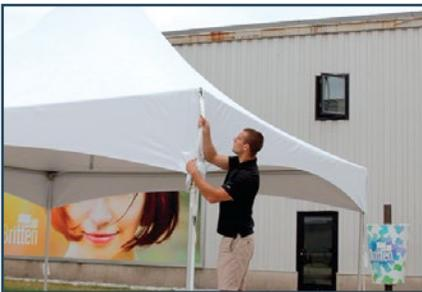
Connect the top carabiner on the outguy strap to the metal loop on the tent bracket.
