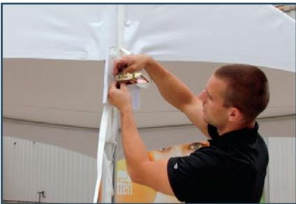
Once the lid is secure, feed the end of the bottom strap up into the ratchet that is located at the bottom end of the top strap (this is the strap installed in step 2).
