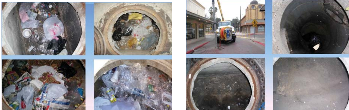
Storm drain manhole before maintenance. Storm drain manhole after maintenance.
