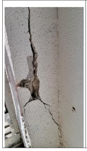
This is located on the fourth floor and accessible through the condo unit at the lanai. The superficial stucco has cracked substantially, but this is cosmetic only and stucco is not a "primary structural member".
