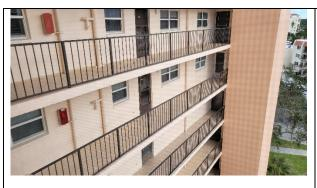
Walkways and balconies may or may not be integrated with the building structure as to be considered a primary structural member. See photo angle below. This example is primary.
