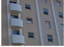
Small balconies independent of the primary building structure. These balconies were constructed after the building was erected.
