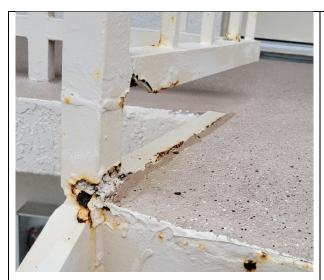
The handrail to the left may need attention, especially if nearby supports are just as deteriorated.
