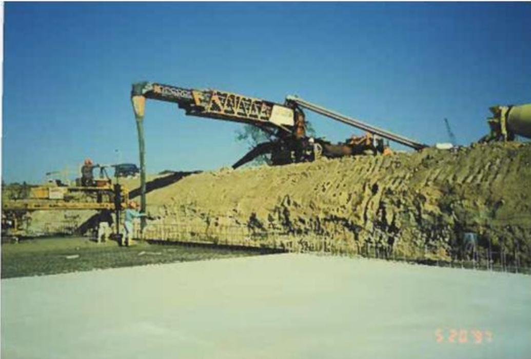
The last piece of equipment to cover is the Belt Conveyor Truck.
