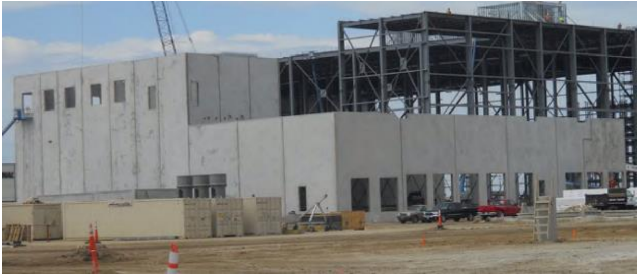
Fig. 2 (from Part 1): Erected tilt-up panels placed side-by-side
