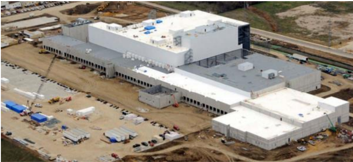
Fig. 1 (from Part 1): Progress photo of a project with tilt-up concrete walls
