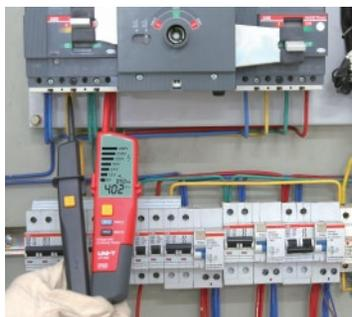
UT18 series are designed for testing AC/DC voltage, 3-phase voltage, phase sequence, continuity, and more. This series is categorized as CAT IV 600V and meets IP65 standard. These voltage testers are perfect tools for electricians to quickly measure voltage levels in all environments. This series should NOT be used with 110V electrical systems.
