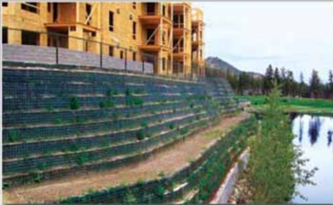
Wall face using Mechanically Stabilized Earth (MSE) technology
