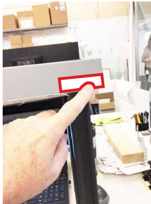
On front or back of ceiling track if hidden under skin (1” overlap needed)
