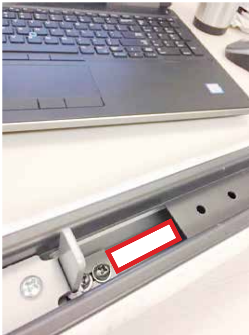
On inside of ceiling track accessible through distribution slot
