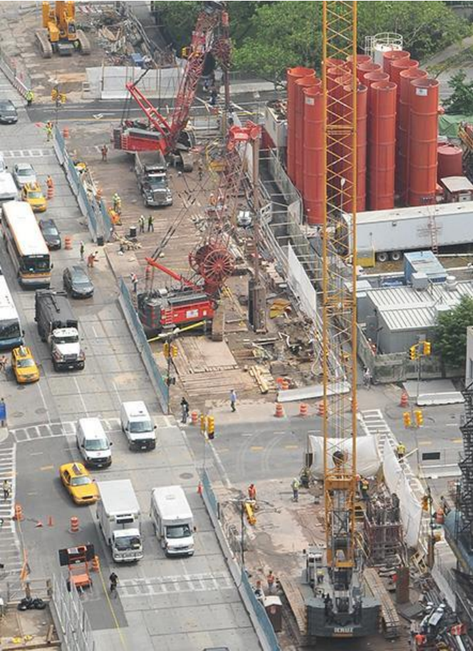
Cut and Cover Station Construction
