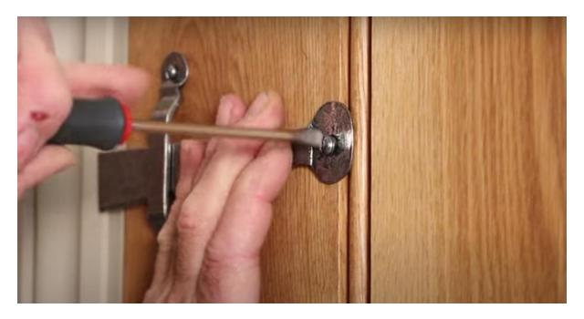
Step 4: Install the Thump Latch Lever Piece
