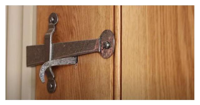
Step 5: Secure the Thumb Latch Handle on the door
