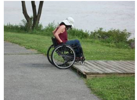
No accessible route is provided to access this boardwalk.
