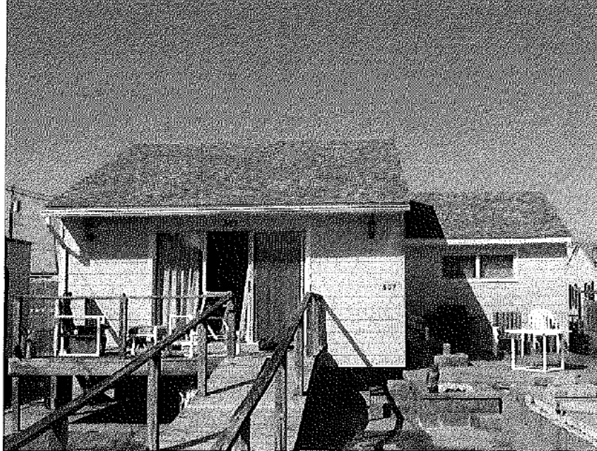
Photograph 1 View of the front (south) side of the subject building.
