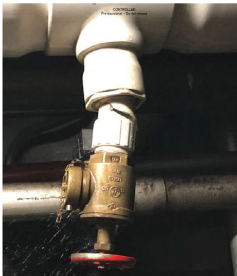
Cracked Low Point Drain
