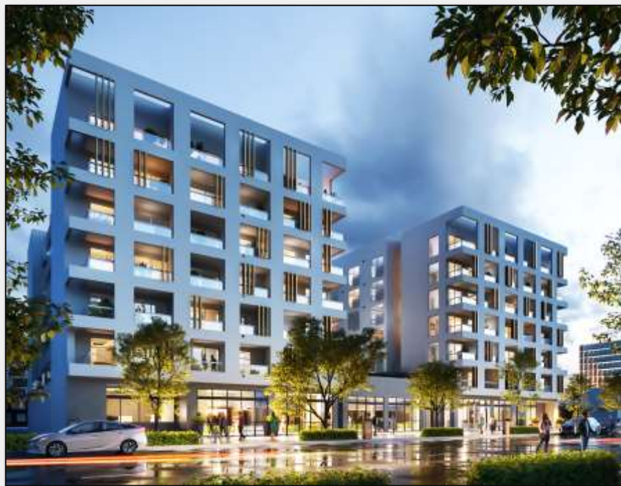
4135 Park Blvd – San Diego, CA – 190 Units, Under Construction - Not a Fund Investment
