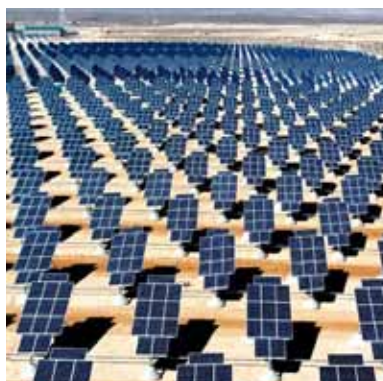
AGUA CALIENTE SOLAR PROJECT Agreed January 2011 US DoE $967 m loan to construct 290 MW solar facility | Maricopa, AZ
