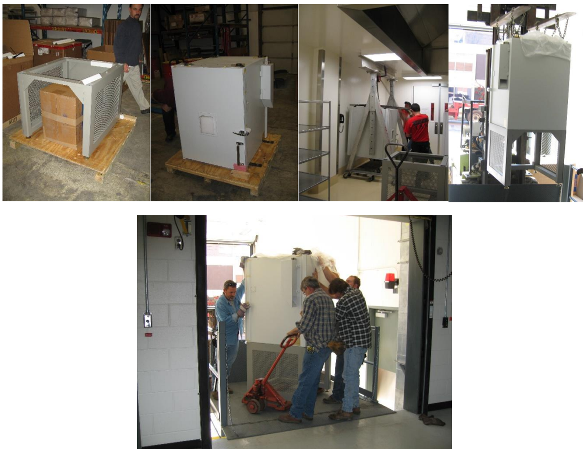
Typical XRAD320 Installation & Rigger Operations
