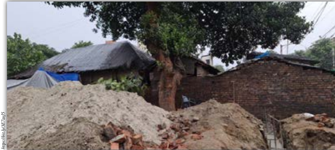
New temple construction work begins at Srila Prabhupada's birthplace in Tollygunge, Kolkata, as the land was recently acquired by ISKCON
