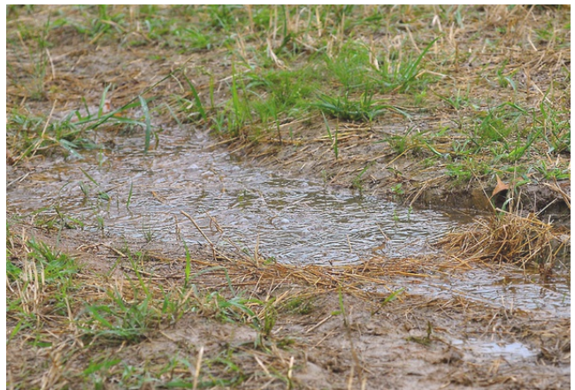
Water pooling in yard; recommend drainage
