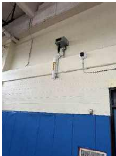
Electric Steam Humidifier Retrofit to Serve Gymnasium (left, middle) and Gymnasium Return Grille (right)
