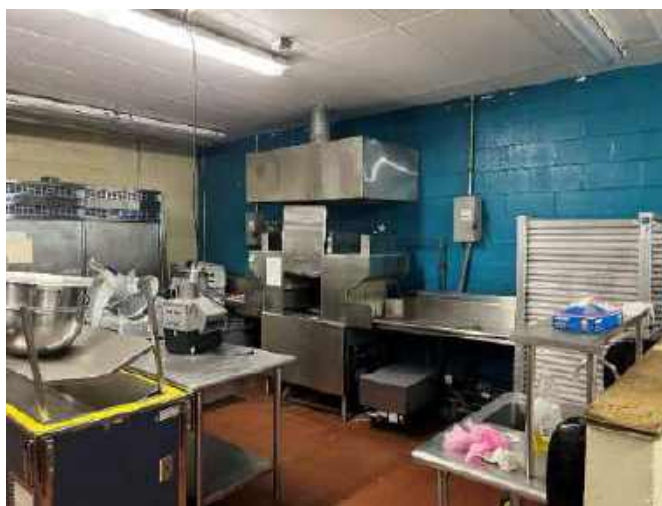
Dishwasher Type II Exhaust Hood
