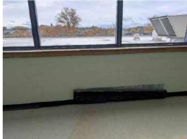
Detached Perimeter Electric Baseboard Heating in Corridors
