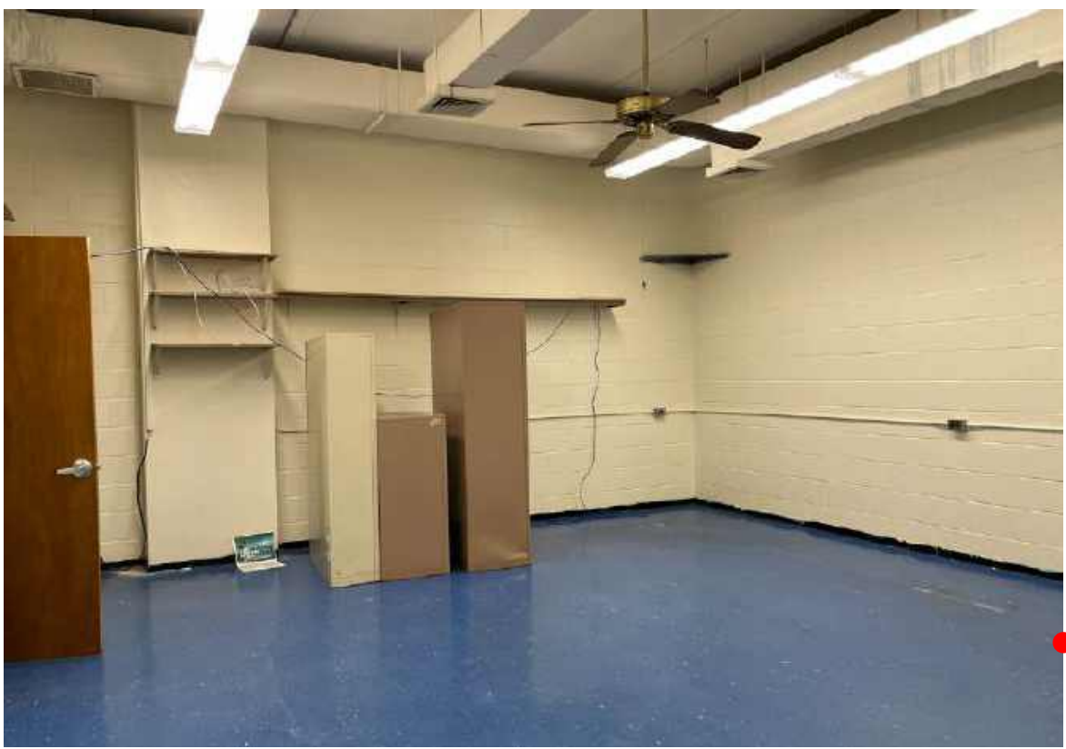
Classroom with no windows
