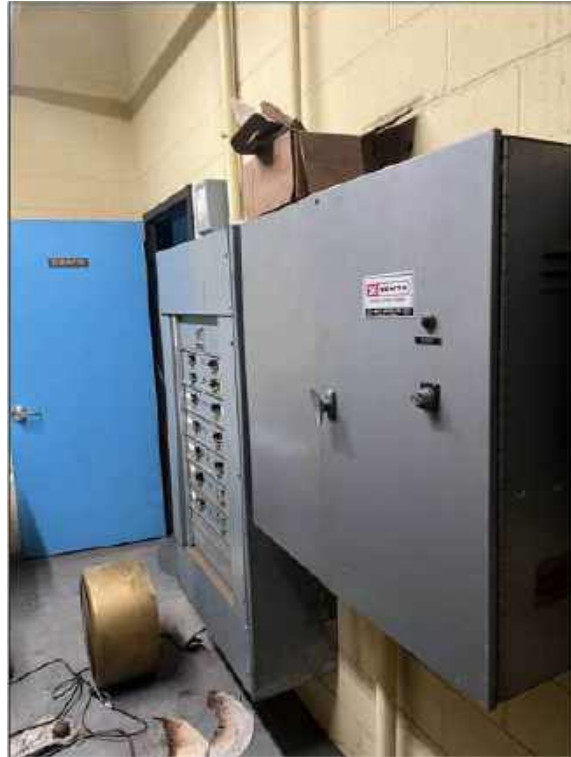
Existing 75kW Natural Gas Kohler Generator, EDP and Zenith ATS
