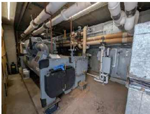
Carrier Evergreen Water Cooled Chiller
