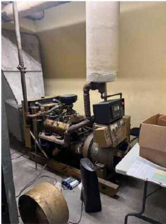
Existing 75kW Natural Gas Kohler Generator, EDP and Zenith ATS
