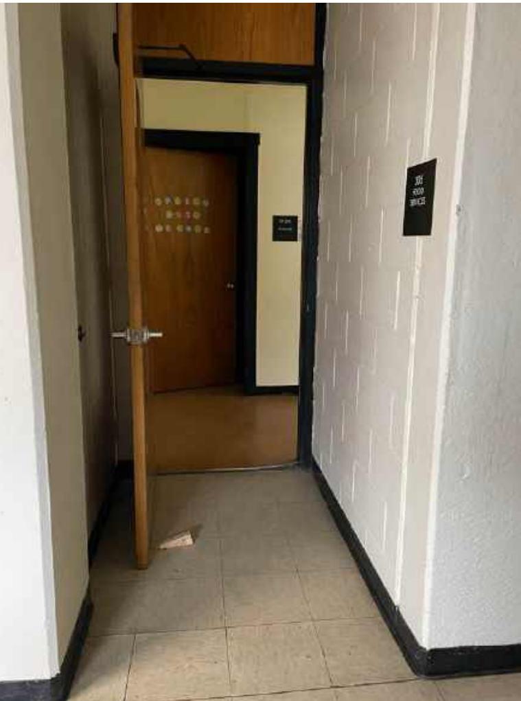
Door Alcoves with no maneuvering clearance
