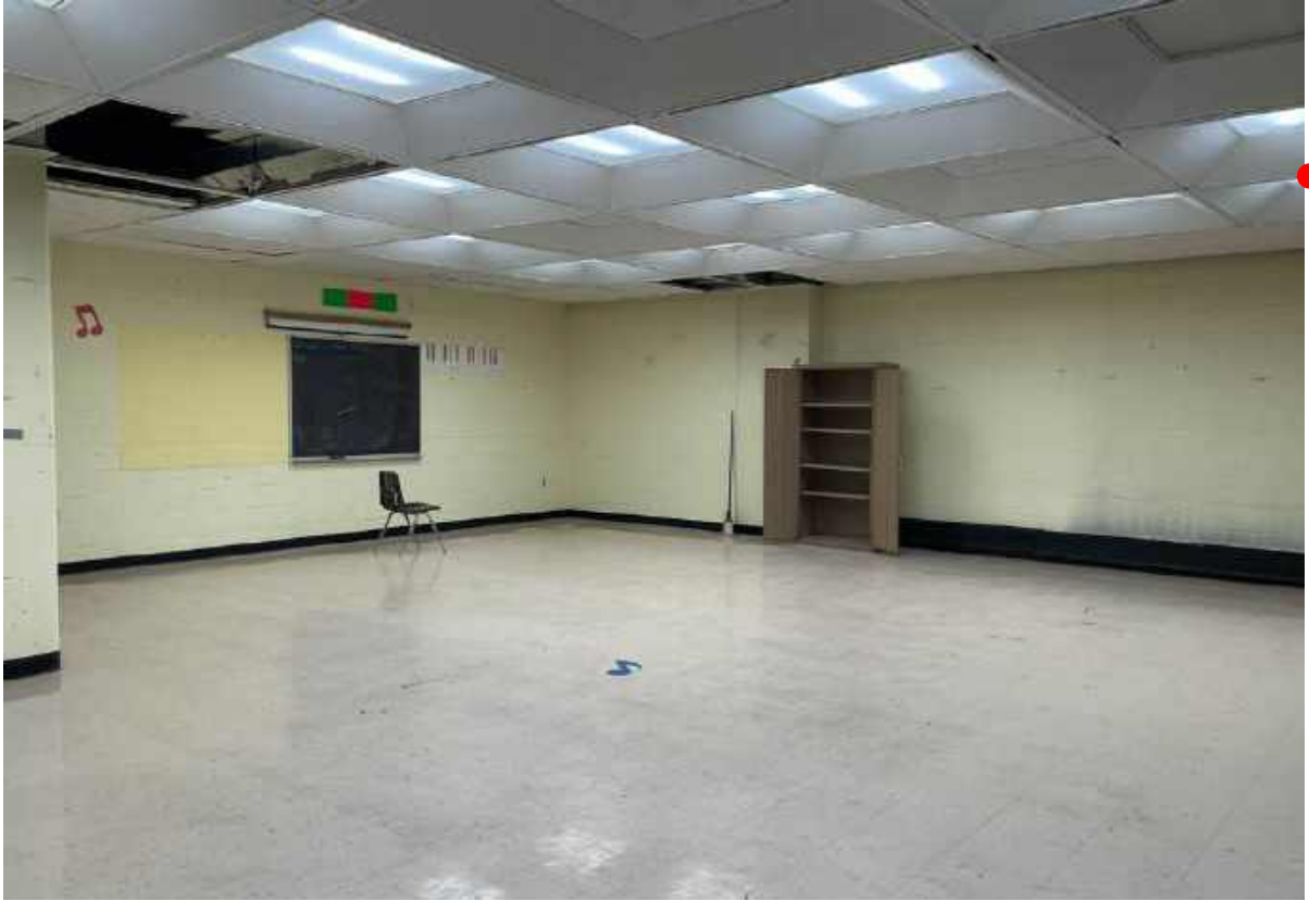
Classroom with no windows
