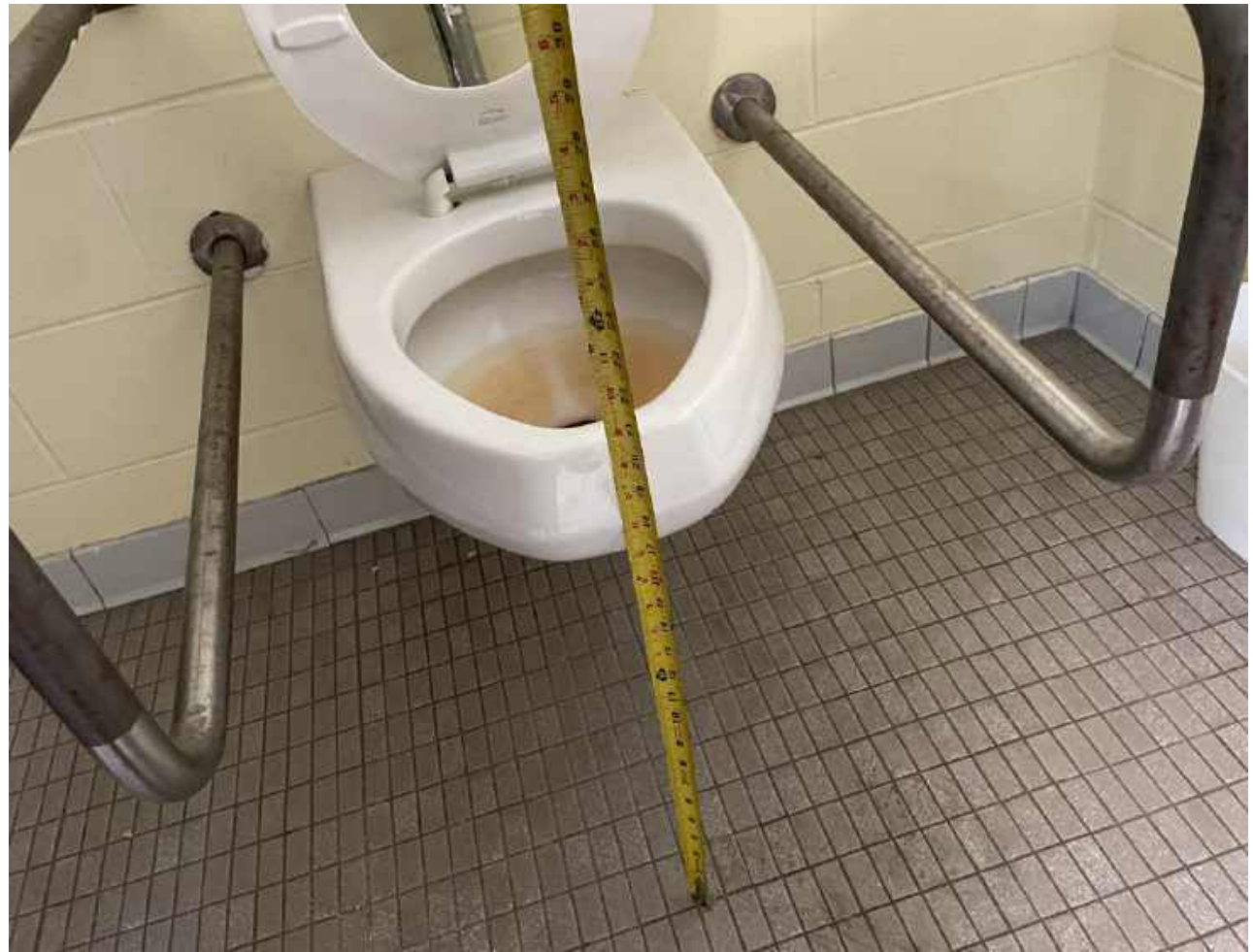
Water Closet - mounted to high
