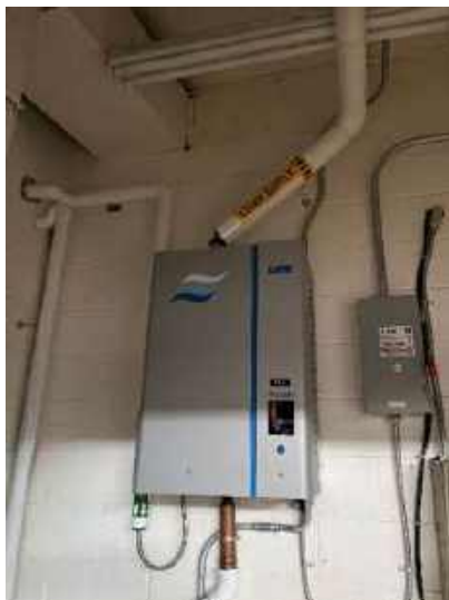
Electric Steam Humidifier Retrofit to Serve Gymnasium (left, middle) and Gymnasium Return Grille (right)
