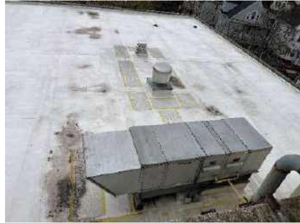
Gas-Fired Heating Only RTUs and Exhaust Fans on Lower Gym Roof
