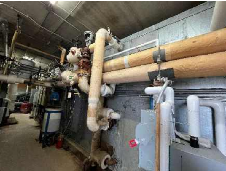
AHU-1 (left) and Electric Steam Humidifier Retrofitted to AHU-1 (right)
