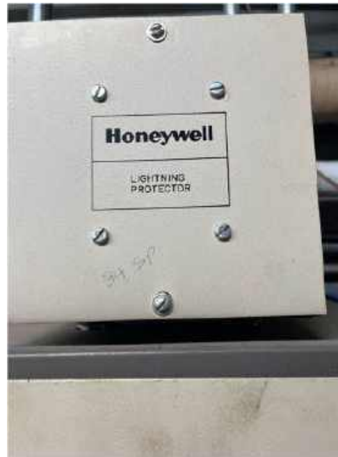
Lightning Protection Control Equipment in Penthouse
