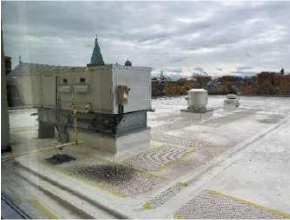
Gas-Fired Heating Only RTUs and Exhaust Fans on Lower Gym Roof
