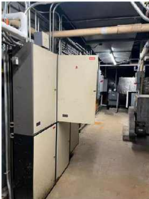
Lightning Protection Control Equipment in Penthouse
