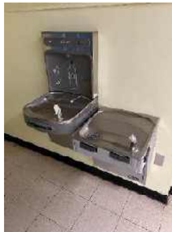
Water Cooler with Bottle Filler
