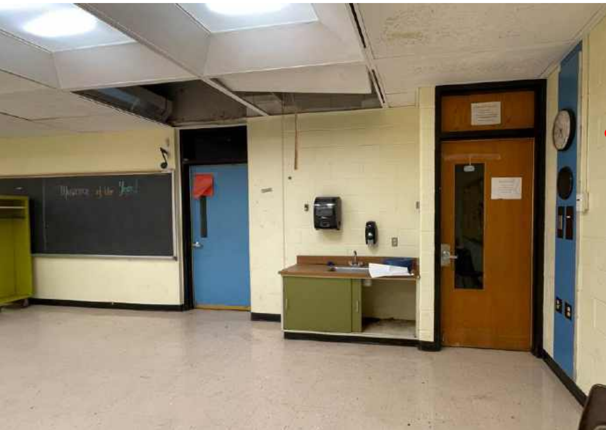
Classroom with no windows
