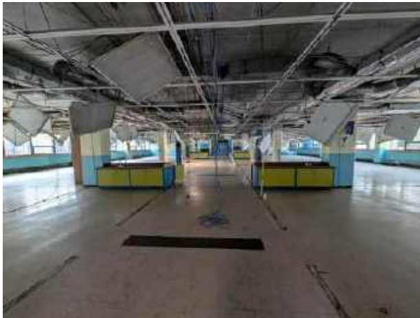
Classroom Wing with Interior Walls Removed, Common Plenum Return, and Linear Diffusers for Ventilation along Central Corridor (left) and Linear Diffusers along Classroom Perimeter (right)
