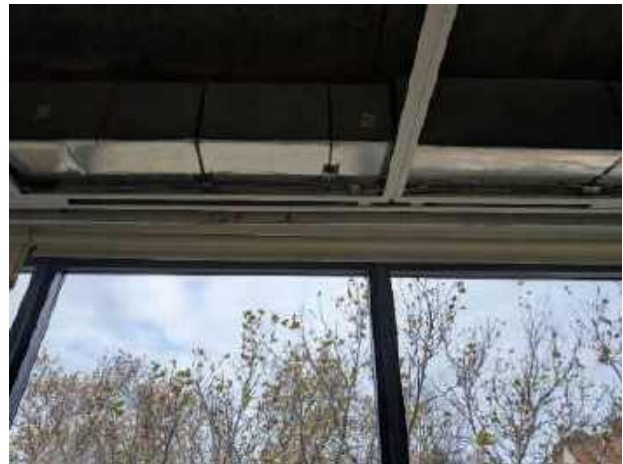
Classroom Wing with Interior Walls Removed, Common Plenum Return, and Linear Diffusers for Ventilation along Central Corridor (left) and Linear Diffusers along Classroom Perimeter (right)
