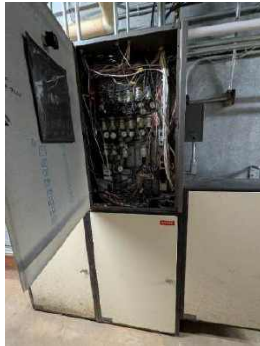
Honeywell Pneumatic Controllers
