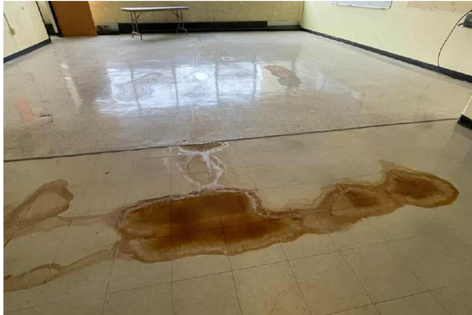
Leak in roof
