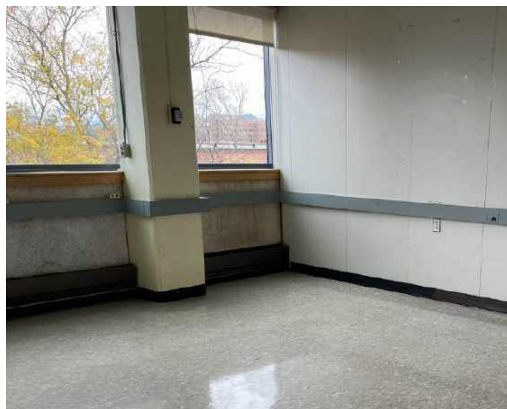
Tectum panels on exterior wall
