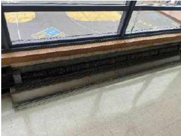
Detached Perimeter Electric Baseboard Heating in Corridors
