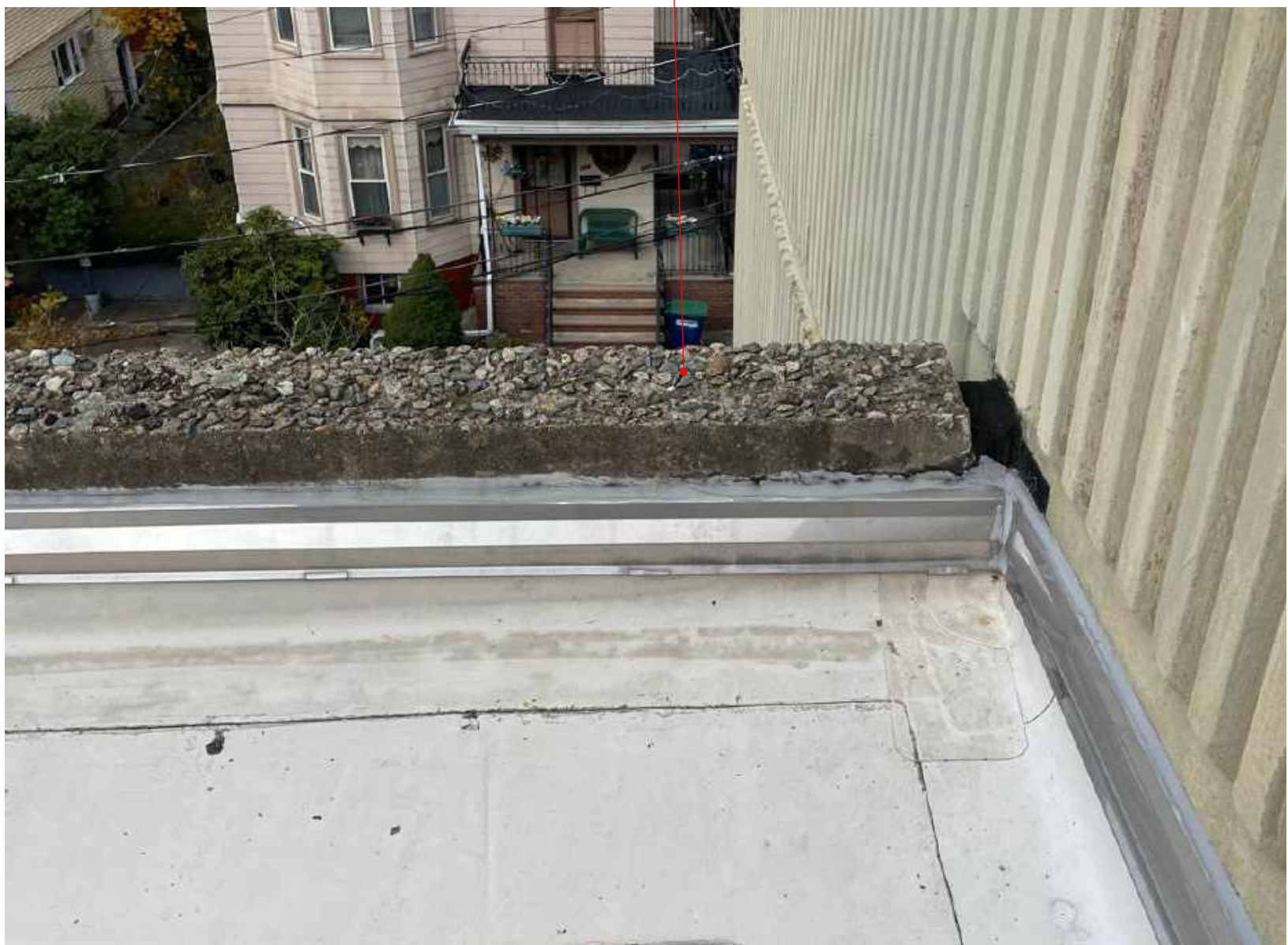
Deteriorating parapet
