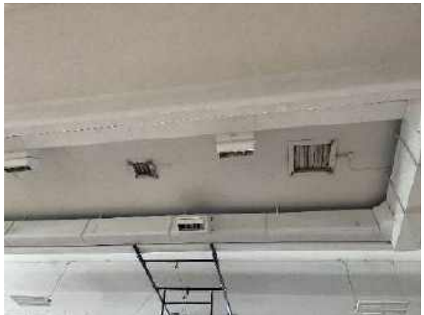
Gymnasium Supply Ductwork and Exhaust Louver
