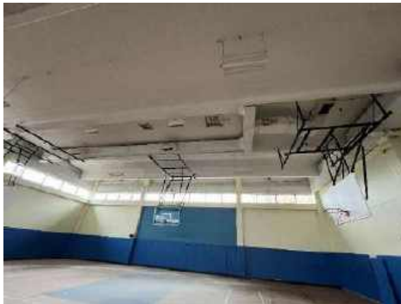
Gymnasium Supply Ductwork and Exhaust Louver
