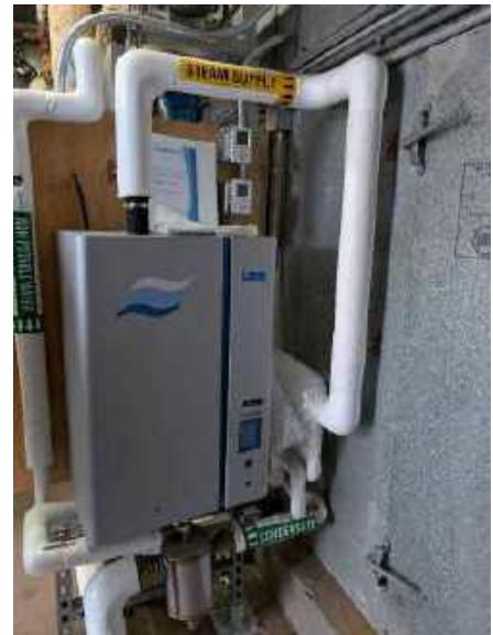
AHU-1 (left) and Electric Steam Humidifier Retrofitted to AHU-1 (right)
