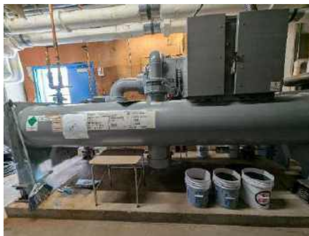
Carrier Evergreen Water Cooled Chiller
