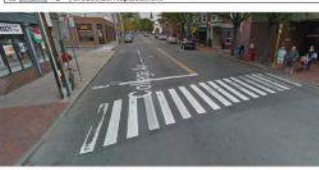
FIGURE 5: COLLEGE AVENUE CROSSING (FACING NORTH)
