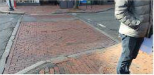
FIGURE 15.3: CROSSING AT ELM STREET (FACING WEST)
