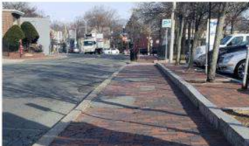
FIGURE 16.2: SOUTH SIDEWALK AT GROVE STREET (FACING EAST)
