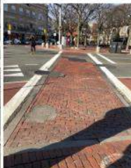
FIGURE 6: COLLEGE AVENUE CROSSING II (FACING WEST)
