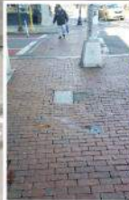
FIGURE 9.1: DOVER STREET CROSSING (FACING NORTH)
