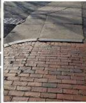
FIGURE 16.1: NORTH SIDEWALK AT GROVE STREET (FACING WEST)
