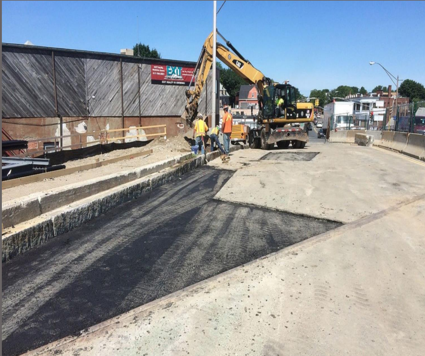
Ball Square Bridge: July 2015
