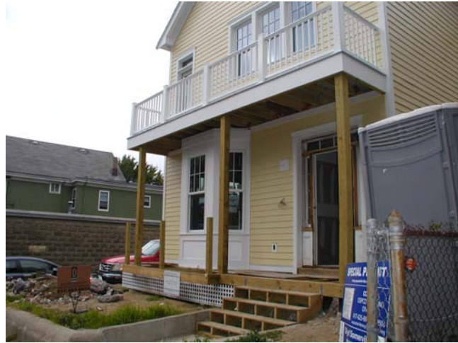
Front façade after construction commenced
