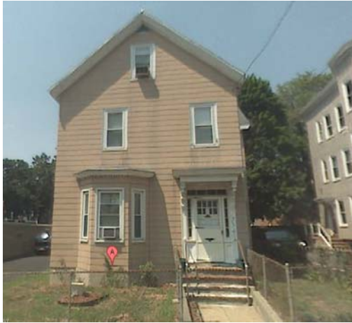
Front façade before renovations
