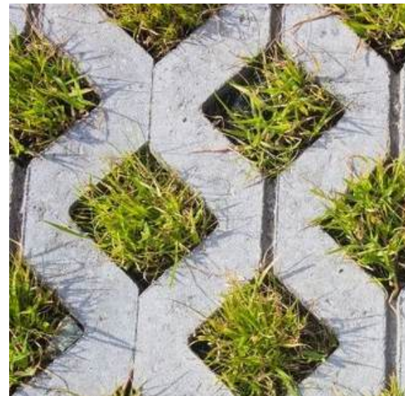
Figure 26 Permeable pavement can consist of a grid- like system that allows water to pass through into the soil. (Image: Billy.com n.d.)
