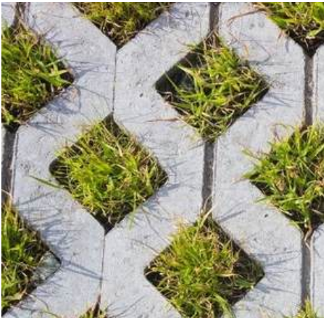
Figure 14. Permeable pavement can consist of a grid-like system that allows water to pass through into the soil. (Image: Billy.com n.d.)
