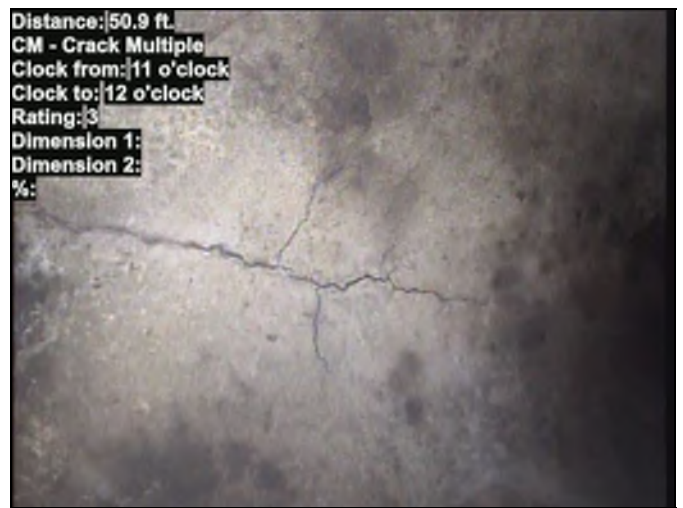
Distance: 50.9 ft. CM - Crack Multiple Clock from: 11 o'clock Clock to: 12 o'clock Rating: 3 Dimension 1: Dimension 2: %: Photo: 666667947.00-22084.00-20240421-205127-205651.JPG At: 50.9 ft. CM - Crack Multiple 11/12 Joint: No
