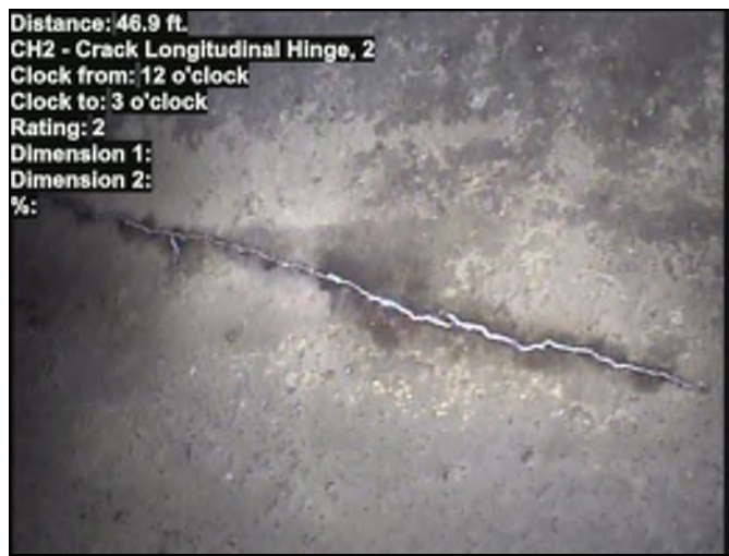
Photo: 22084.00-22283.00-20240421-222809-223140.JPG At: 46.9 ft. 12/3 CH2 - Crack Longitudinal Hinge, 2 Joint: No
