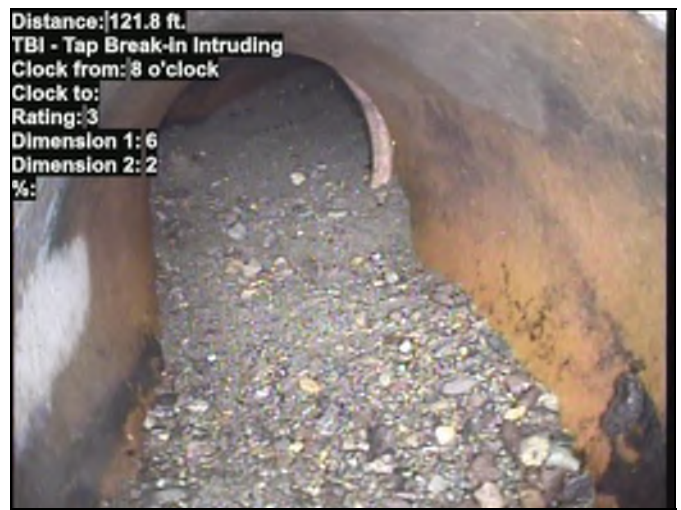
Distance: 121.8 ft. TBI - Tap Break-in Intruding Clock from: 8 o'clock Clock to: Rating: 3 Dimension 1: 6 Dimension 2: 2 %: Photo: 666667947.00-22084.00-20240421-205127-210016.JPG At: 121.8 ft. 8/. TBI - Tap Break-in Intruding Joint: No
