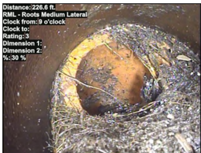
Distance: 226.6 ft. RML - Roots Medium Lateral Clock from: 9 o'clock Clock to: Rating: 3 Dimension 1: Dimension 2: %: 30 % Photo: 666667978.00-30328.00-20240422-010742-012341.JPG At: 226.6 ft. 9/. RML - Roots Medium Lateral Joint: No 30 %
