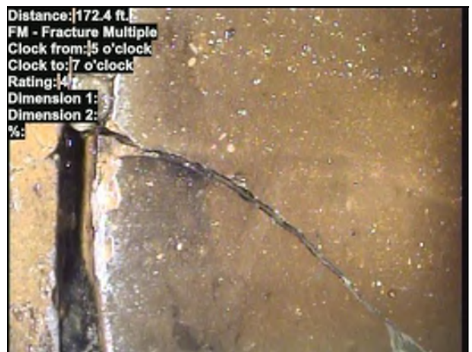
Distance: 172.4 ft. FM - Fracture Multiple Clock from: 5 o'clock Clock to: 7 o'clock Rating: 4 Dimension 1: Dimension 2: %: Photo: 666667978.00-30328.00-20240422-010742-012041.JPG At: 172.4 ft. 5/7 FM - Fracture Multiple Joint: No
