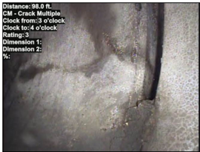
Distance: 98.0 ft. CM - Crack Multiple Clock from: 3 o'clock Clock to: 4 o'clock Rating: 3 Dimension 1: Dimension 2: %: Photo: 666667947.00-22084.00-20240421-205127-205907.JPG At: 98 ft. 3/4 CM - Crack Multiple Joint: No
