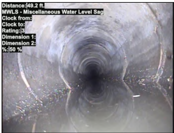
Distance: 49.2 ft. MWLS - Miscellaneous Water Level Sag Clock from: Clock to: Rating: 3 Dimension 1: Dimension 2: %: 50 % Photo: 666667947.00-22084.00-20240421-205127-205641.JPG At: 49.2 ft. MWLS - Miscellaneous Water Level Sag Joint: No 50 %
