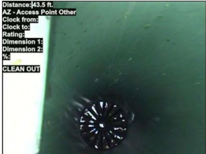
Photo: SW-CB-03622-32-6424-20230905-082128.JPG At: 43.5 ft. AZ - Access Point Other Joint: No CLEAN OUT
