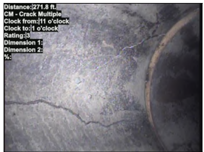
Distance: 271.8 ft. CM - Crack Multiple Clock from: 11 o'clock Clock to: 1 o'clock Rating: 3 Dimension 1: Dimension 2: %: Photo: 22084.00-22283.00-20240421-222809-224031.JPG At: 271.8 ft. CM - Crack Multiple 11/1 Joint: No
