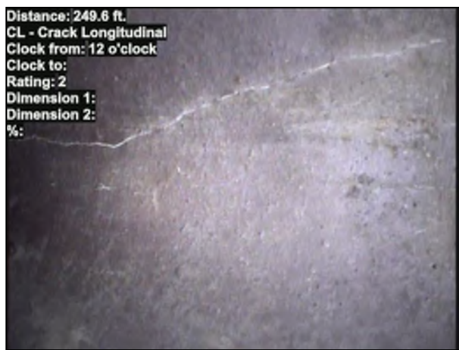
Distance: 249.6 ft. CL - Crack Longitudinal Clock from: 12 o'clock Clock to: Rating: 2 Dimension 1: Dimension 2: %: Photo: 22084.00-22283.00-20240421-222809-223944.JPG At: 249.6 ft. 12/. CL - Crack Longitudinal Joint: No
