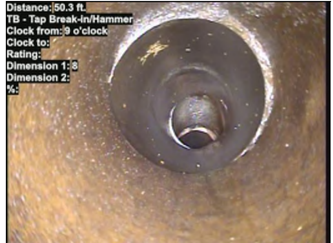
Distance: 50.3 ft. TB - Tap Break-in/Hammer Clock from: 9 o'clock Clock to: Rating: Dimension 1: 8 Dimension 2: %: Photo: 666667978.00-30328.00-20240422-010742-011218.JPG At: 50.3 ft. 9/. TB - Tap Break-in/Hammer Joint: No
