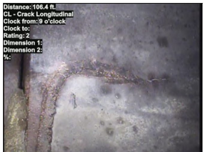
Photo: 22084.00-22283.00-20240421-222809-223403.JPG At: 106.4 ft. 9/. CL - Crack Longitudinal Joint: No
