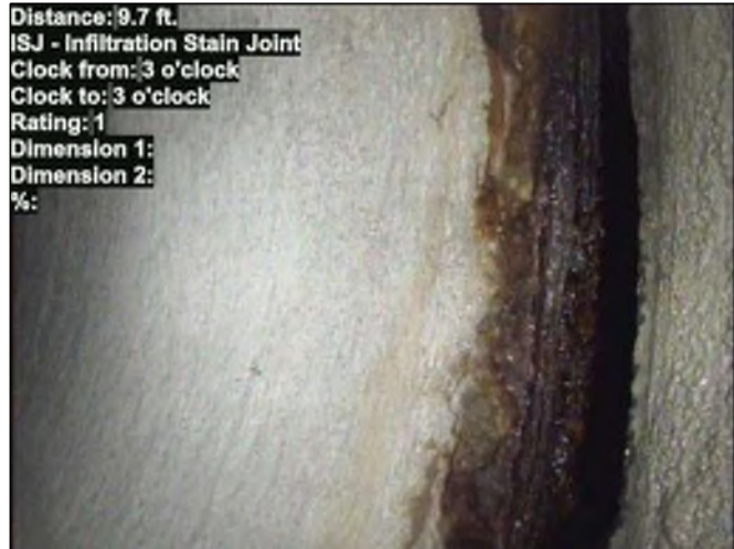
Photo: 32-6444-32-6443-20230905-105823.JPG At: 9.7 ft. 3/3 ISJ - Infiltration Stain Joint Joint: Yes
