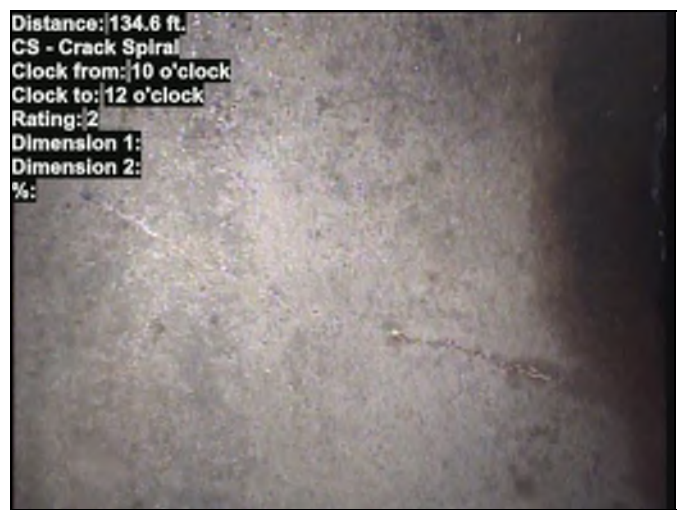
Distance: 134.6 ft. CS - Crack Spiral Clock from: 10 o'clock Clock to: 12 o'clock Rating: 2 Dimension 1: Dimension 2: %: Photo: 666667947.00-22084.00-20240421-205127-210108.JPG At: 134.6 ft. CS - Crack Spiral 10/12 Joint: No
