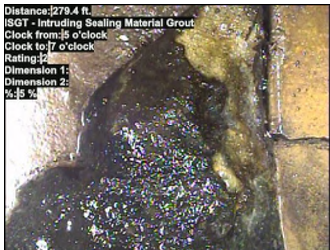
Distance: 279.4 ft. ISGT - Intruding Sealing Material Grout Clock from: 5 o'clock Clock to: 7 o'clock Rating: 2 Dimension 1: Dimension 2: %: 5 % Photo: 666667978.00-30328.00-20240422-010742-012724.JPG At: 279.4 ft. 5/7 ISGT - Intruding Sealing Material Grout Joint: No 5 %
