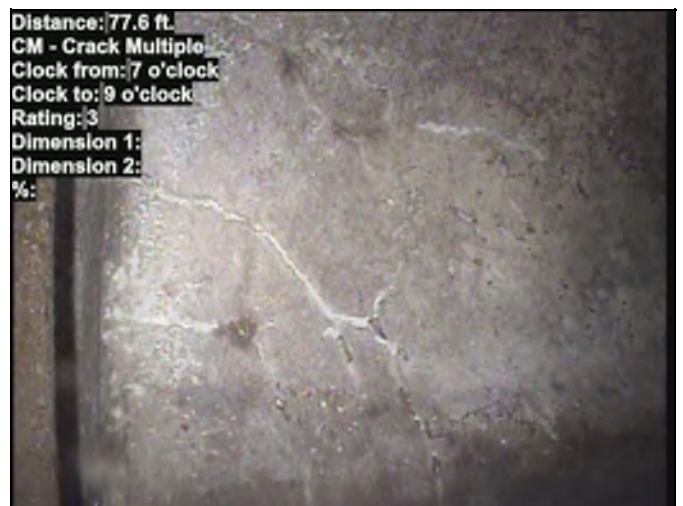
Distance: 77.6 ft. CM - Crack Multiple Clock from: 7 o'clock Clock to: 9 o'clock Rating: 3 Dimension 1: Dimension 2: %: Photo: 666667947.00-22084.00-20240421-205127-205821.JPG At: 77.6 ft. 7/9 CM - Crack Multiple Joint: No
