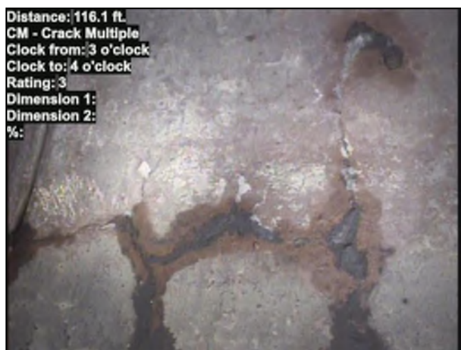
Photo: 22084.00-22283.00-20240421-222809-223430.JPG At: 116.1 ft. 3/4 CM - Crack Multiple Joint: No
