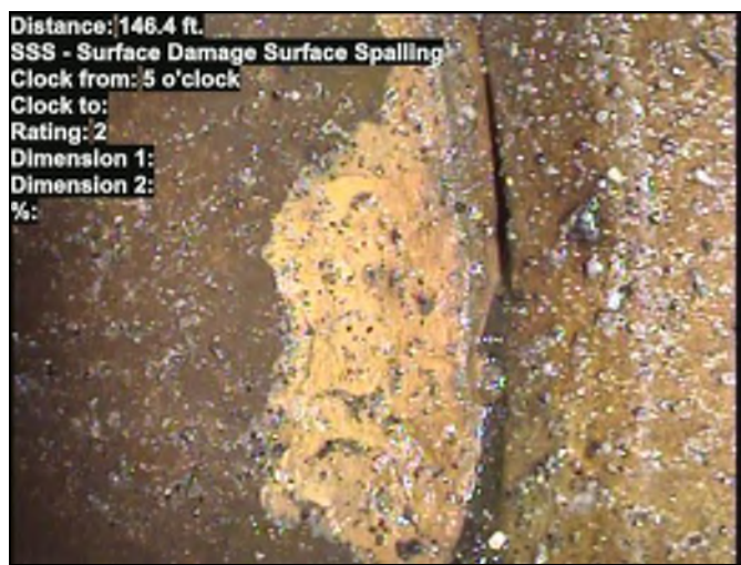
Distance: 146.4 ft. SSS - Surface Damage Surface Spalling Clock from: 5 o'clock Clock to: Rating: 2 Dimension 1: Dimension 2: %: Photo: 666667978.00-30328.00-20240422-010742-011853.JPG At: 146.4 ft. 5/. SSS - Surface Damage Surface Spalling Joint: No
