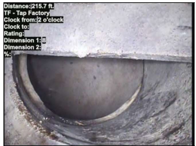
Distance: 215.7 ft. TF - Tap Factory Clock from: 2 o'clock Clock to: Rating: Dimension 1: 8 Dimension 2: %: Photo: 22084.00-22283.00-20240421-222809-223845.JPG At: 215.7 ft. 2/. TF - Tap Factory Joint: No
