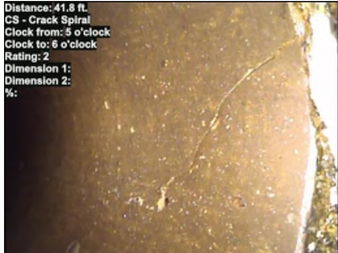
Distance: 41.8 ft. CS - Crack Spiral Clock from: 5 o'clock Clock to: 6 o'clock Rating: 2 Dimension 1: Dimension 2: %: Photo: 666667978.00-30328.00-20240422-010742-011148.JPG At: 41.8 ft. 5/6 CS - Crack Spiral Joint: No
