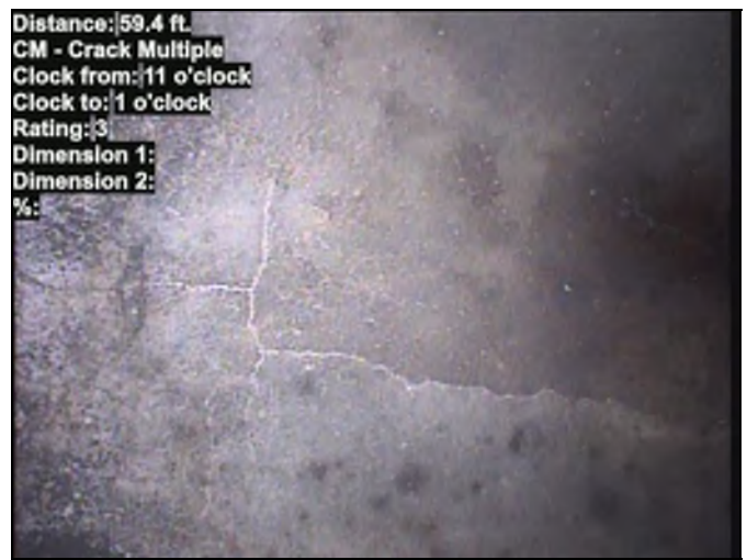
Photo: 22084.00-22283.00-20240421-222809-223210.JPG At: 59.4 ft. 11/1 CM - Crack Multiple Joint: No
