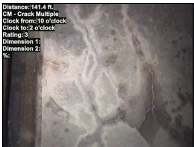
Distance: 141.4 ft. CM - Crack Multiple Clock from: 10 o'clock Clock to: 2 o'clock Rating: 3 Dimension 1: Dimension 2: %: Photo: 666667947.00-22084.00-20240421-205127-210133.JPG At: 141.4 ft. CM - Crack Multiple 10/2 Joint: No
