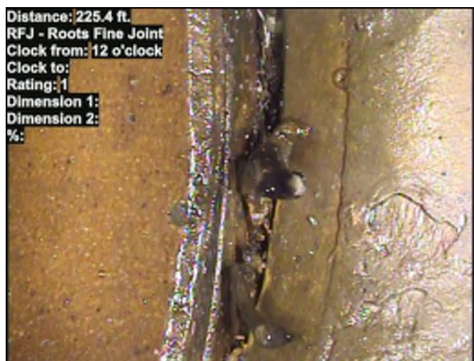
Distance: 225.4 ft. RFJ - Roots Fine Joint Clock from: 12 o'clock Clock to: Rating: 1 Dimension 1: Dimension 2: %: Photo: 666667978.00-30328.00-20240422-010742-012312.JPG At: 225.4 ft. 12/. RFJ - Roots Fine Joint Joint: Yes
