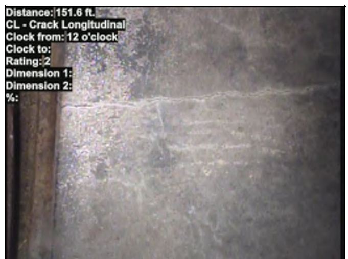
Distance: 151.6 ft. CL - Crack Longitudinal Clock from: 12 o'clock Clock to: Rating: 2 Dimension 1: Dimension 2: %: Photo: 666667947.00-22084.00-20240421-205127-210208.JPG At: 151.6 ft. 12/. CL - Crack Longitudinal Joint: No
