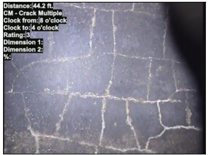
Distance: 44.2 ft. CM - Crack Multiple Clock from: 8 o'clock Clock to: 4 o'clock Rating: 3 Dimension 1: Dimension 2: %: Photo: 666667947.00-22084.00-20240421-205127-205608.JPG At: 44.2 ft. 8/4 CM - Crack Multiple Joint: No
