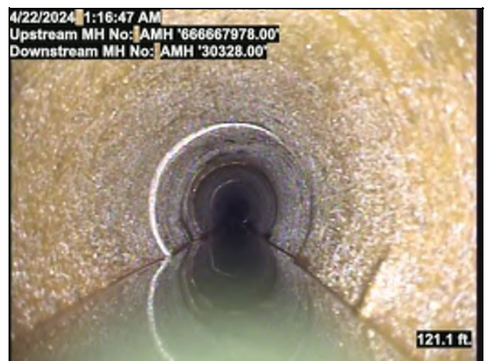
4/22/2024 1:16:47 AM Upstream MH No: AMH '666667978.00' Downstream MH No: AMH '30328.00' Photo: 666667978.00-30328.00-20240422-010742-011645.JPG At: 120.1 ft. RFJ - Roots Fine Joint 12/12 Joint: Yes
