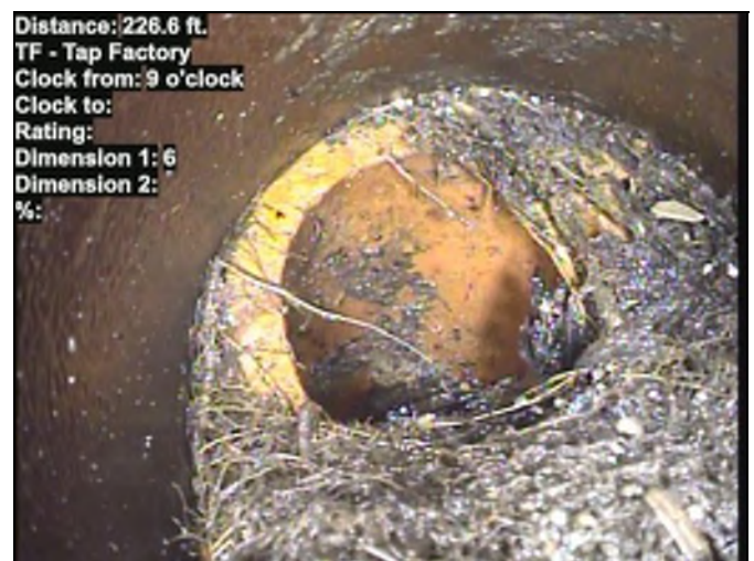
Distance: 226.6 ft. TF - Tap Factory Clock from: 9 o'clock Clock to: Rating: Dimension 1: 6 Dimension 2: %: Photo: 666667978.00-30328.00-20240422-010742-012331.JPG At: 226.6 ft. 9/. TF - Tap Factory Joint: No
