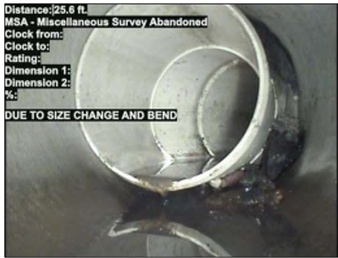
Photo: 32-6421-32-6424-20230905-080056.JPG At: 25.6 ft. MSA - Miscellaneous Survey Abandoned Joint: No DUE TO SIZE CHANGE AND BEND
