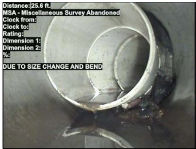
Photo: 32-6421-32-6424-20230905-080056.JPG At: 25.6 ft. MSA - Miscellaneous Survey Abandoned Joint: No DUE TO SIZE CHANGE AND BEND
