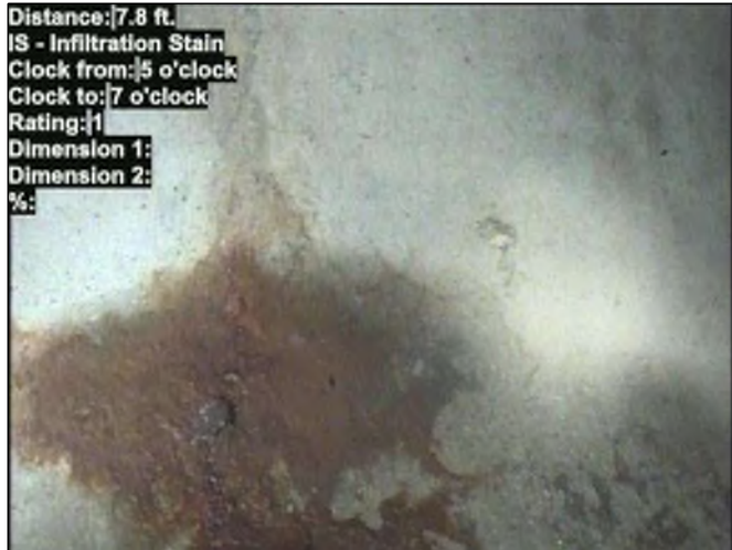
Photo: 32-6421-32-6424-20230905-075303.JPG At: 7.8 ft. 5/7 IS - Infiltration Stain Joint: No
