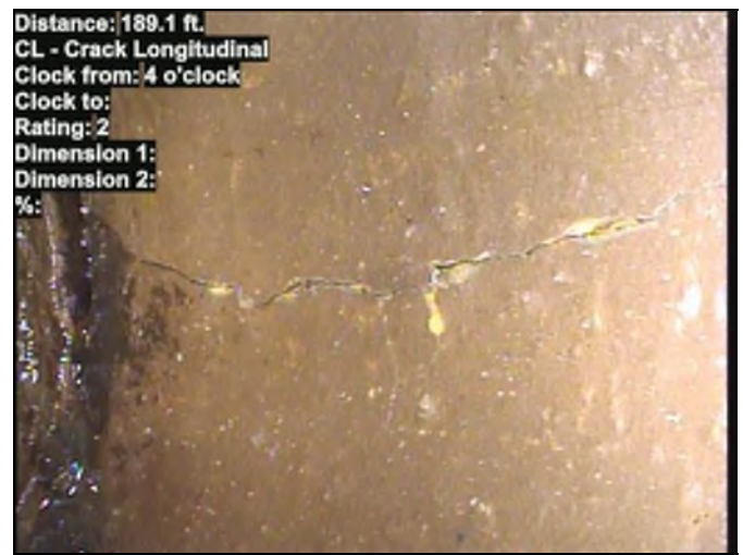
Distance: 189.1 ft. CL - Crack Longitudinal Clock from: 4 o'clock Clock to: Rating: 2 Dimension 1: Dimension 2: %: Photo: 666667978.00-30328.00-20240422-010742-012141.JPG At: 189.1 ft. 4/. CL - Crack Longitudinal Joint: No
