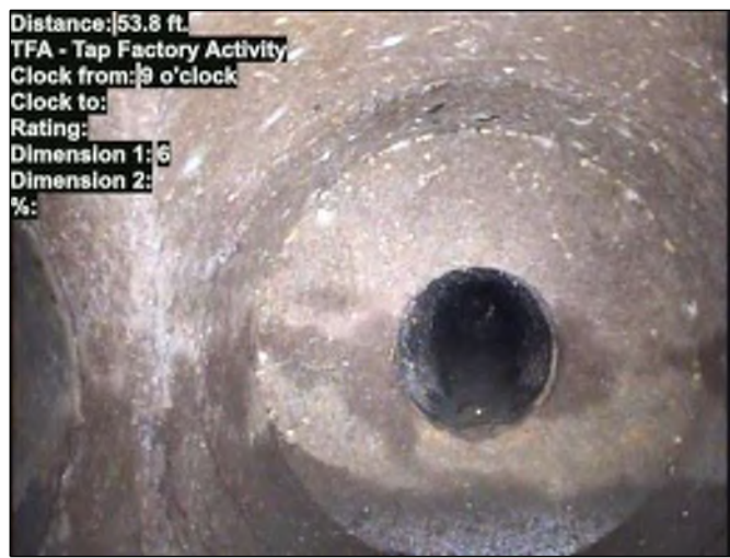
Photo: UNKNOWN-32-6442-20230905-115626.JPG At: 53.8 ft. 9/. TFA - Tap Factory Activity Joint: No
