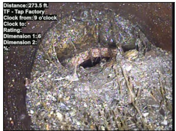
Distance: 273.5 ft. TF - Tap Factory Clock from: 9 o'clock Clock to: Rating: Dimension 1: 6 Dimension 2: %: Photo: 666667978.00-30328.00-20240422-010742-012613.JPG At: 273.5 ft. 9/. TF - Tap Factory Joint: No
