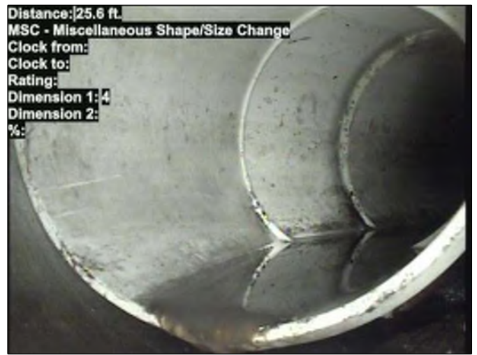
Photo: 32-6421-32-6424-20230905-075823.JPG At: 25.6 ft. MSC - Miscellaneous Shape/Size Change Joint: No
