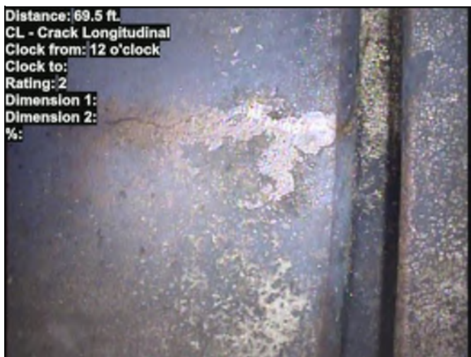
Distance: 69.5 ft. CL - Crack Longitudinal Clock from: 12 o'clock Clock to: Rating: 2 Dimension 1: Dimension 2: %: Photo: 666667947.00-22084.00-20240421-205127-205743.JPG At: 69.5 ft. 12/. CL - Crack Longitudinal Joint: No
