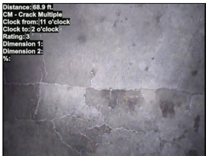
Photo: 22084.00-22283.00-20240421-222809-223236.JPG At: 68.9 ft. 11/2 CM - Crack Multiple Joint: No
