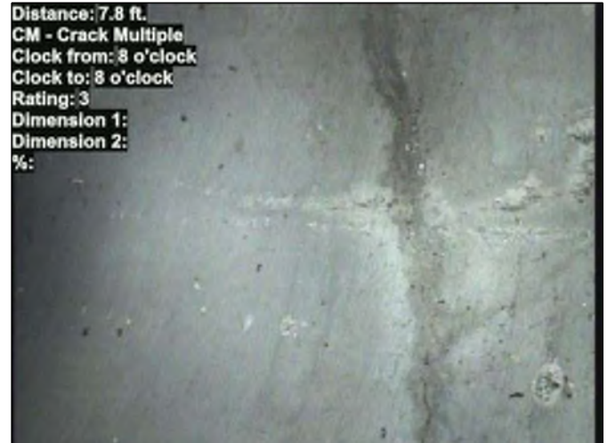
Photo: 32-6421-32-6424-20230905-075244.JPG At: 7.8 ft. 8/8 CM - Crack Multiple Joint: No
