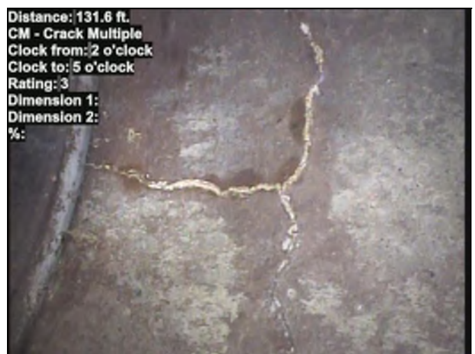
Photo: 22084.00-22283.00-20240421-222809-223504.JPG At: 131.6 ft. 2/5 CM - Crack Multiple Joint: No
