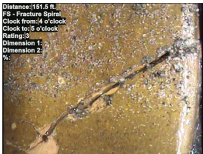
Distance: 151.5 ft. FS - Fracture Spiral Clock from: 4 o'clock Clock to: 5 o'clock Rating: 3 Dimension 1: Dimension 2: %: Photo: 666667978.00-30328.00-20240422-010742-011932.JPG At: 151.5 ft. 4/5 FS - Fracture Spiral Joint: No
