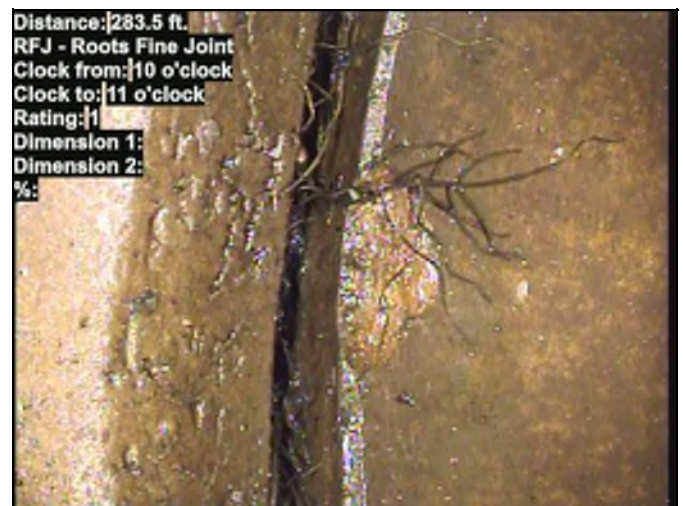
Distance: 283.5 ft. RFJ - Roots Fine Joint Clock from: 10 o'clock Clock to: 11 o'clock Rating: 1 Dimension 1: Dimension 2: %: Photo: 666667978.00-30328.00-20240422-010742-012819.JPG At: 283.5 ft. RFJ - Roots Fine Joint 10/11 Joint: Yes
