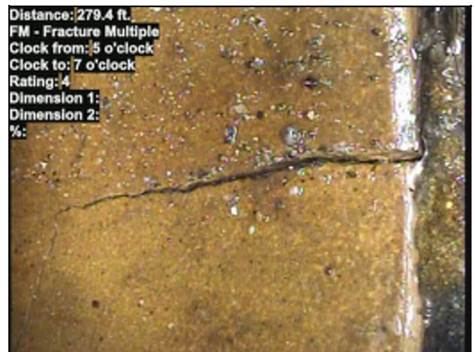
Distance: 279.4 ft. FM - Fracture Multiple Clock from: 5 o'clock Clock to: 7 o'clock Rating: 4 Dimension 1: Dimension 2: %: Photo: 666667978.00-30328.00-20240422-010742-012752.JPG At: 279.4 ft. 5/7 FM - Fracture Multiple Joint: No
