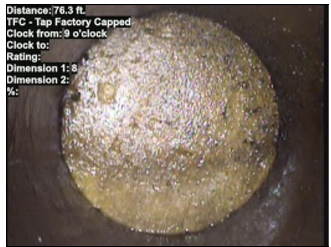
Distance: 76.3 ft. TFC - Tap Factory Capped Clock from: 9 o'clock Clock to: Rating: Dimension 1: 8 Dimension 2: %: Photo: 666667978.00-30328.00-20240422-010742-011408.JPG At: 76.3 ft. 9/. TFC - Tap Factory Capped Joint: No
