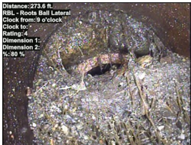
Distance: 273.6 ft. RBL - Roots Ball Lateral Clock from: 9 o'clock Clock to: Rating: 4 Dimension 1: Dimension 2: %: 80 % Photo: 666667978.00-30328.00-20240422-010742-012623.JPG At: 273.6 ft. 9/. RBL - Roots Ball Lateral Joint: No 80 %
