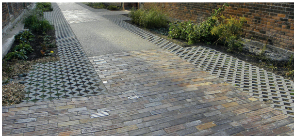
Example alley with plants in Detroit manages stormwater
