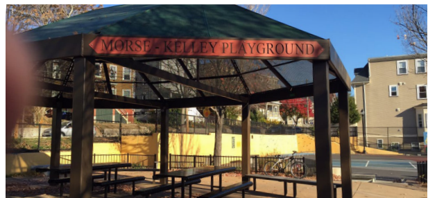
The shade structure in Morse-Kelley Playground
