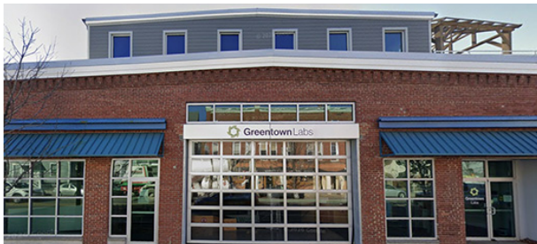
Adaptive re-use with an addition/expansion for a 2nd story
