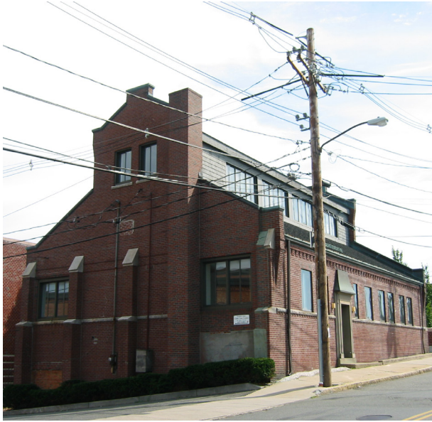
24 Dane Street existing building
