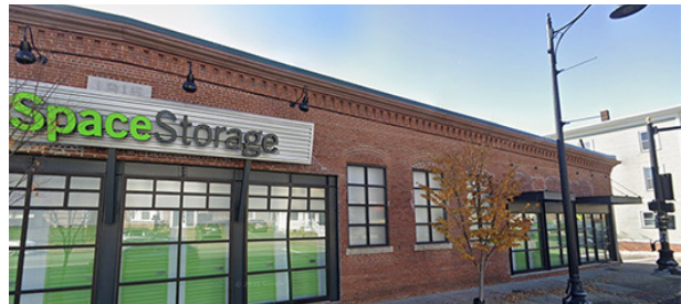
Existing adaptive re-use of an American Tube Works building
