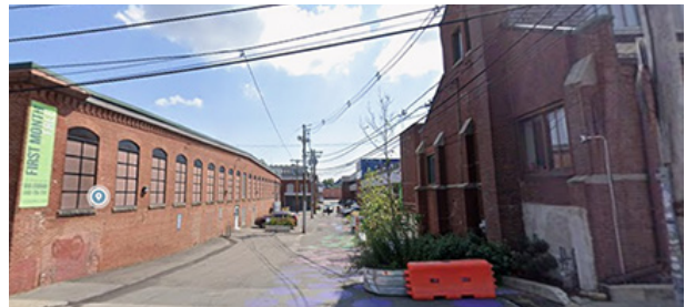
Existing Frost Alley
