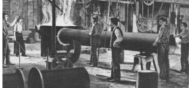
Welding flanges on a steel pipe, circa 1897
