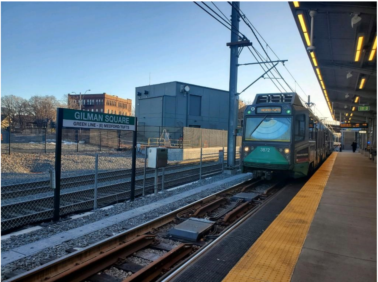
Gilman Square MBTA Station Photo by Rie Lowenstein
