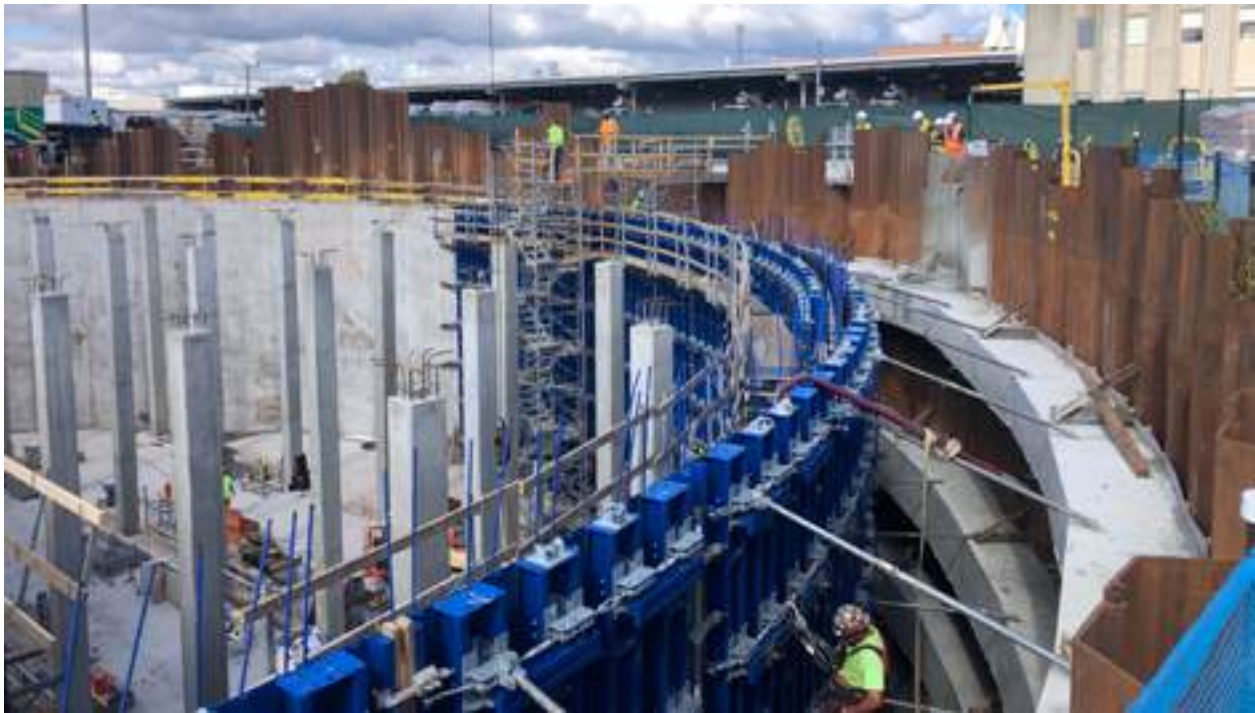
Large stormwater storage tank under construction at the Poplar Street Pump Station. A park will be built above the tank when it is complete.
