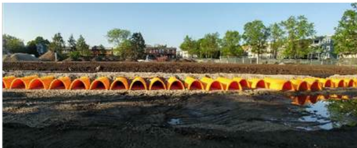
An intricate subsurface stormwater collection system sits below Lincoln Park's athletic fields to alleviate flooding.
