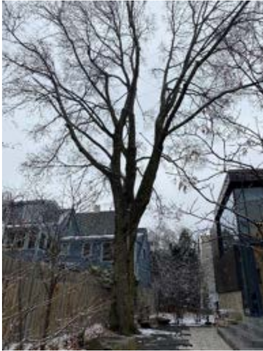
Norway Maple #40894, showing potential targets including seating area, residential sites and new glass library addition
