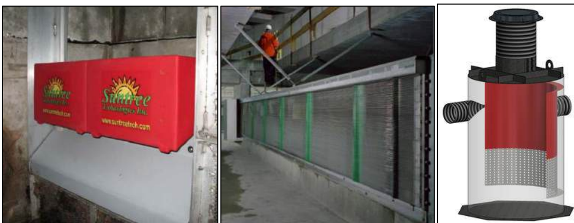
Figure 5 – Dynamic Baffle (Left), Mechanically Cleaned Screen (Center), and Hydrodynamic Separator (Right); Source: OWEA Annual Conference 2010, Options for Solids and Floatables Control
