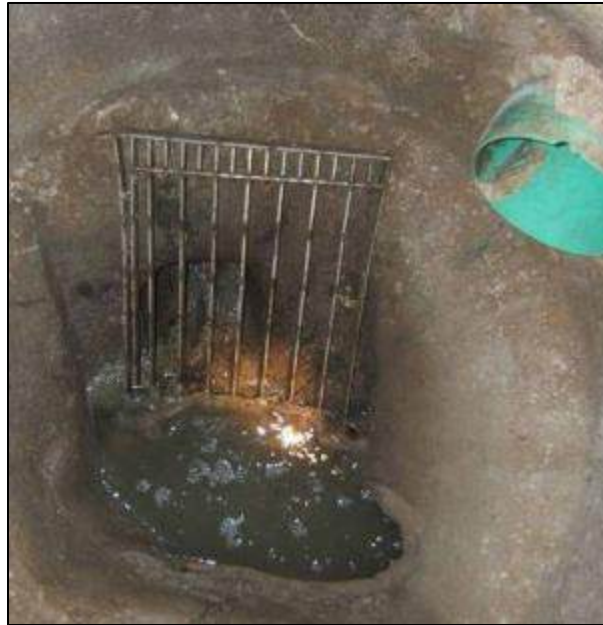
Figure 4 – Example bar screen installation within a combined sewer system manhole; Source: OWEA Annual Conference 2010, Options for Solids and Floatables Control
