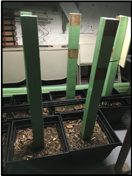
FENCE POSTS & BASES (PLANTERS). 4X4 POSTS (3-1/2" X 3-1/2") SECURED WITH SOIL. OVERALL DIMENSIONS: 17-1/2" (L) 17-1/2" (W) 49" (H)
