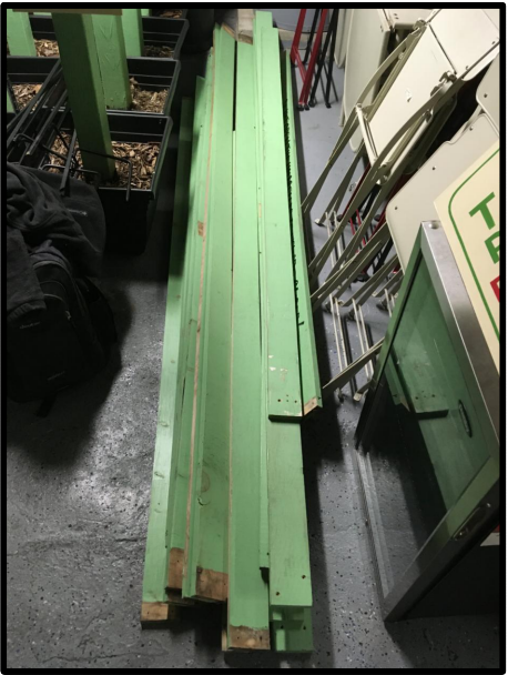
FENCE HORIZONTAL RAILINGS 1X6 LUMBER (3/4" X 5-1/2")
