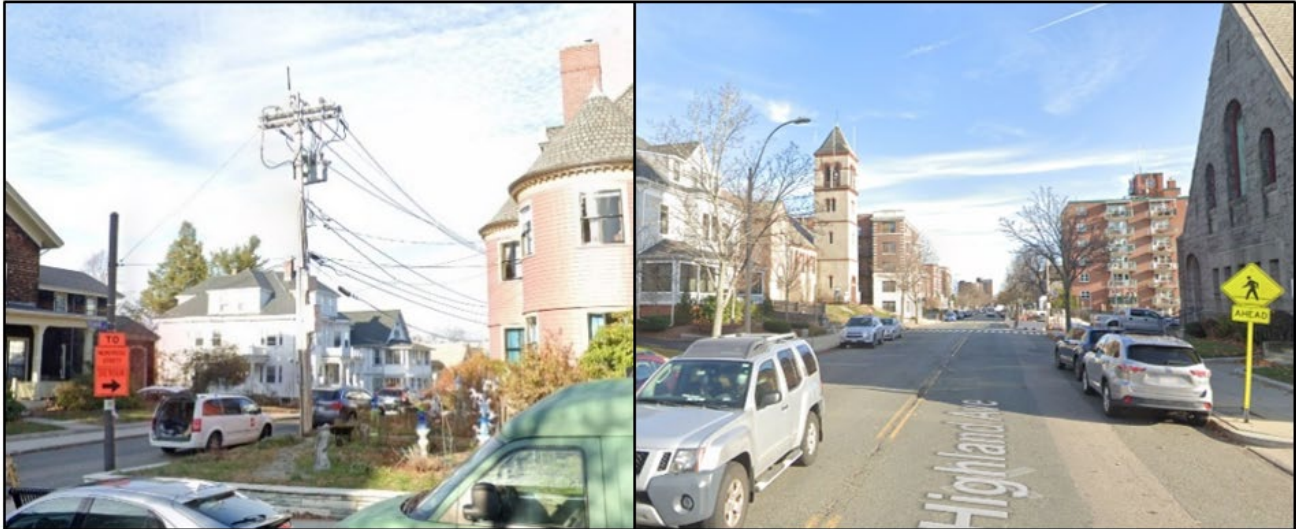
Figure 3-2. Typical streets in Somerville. (Left) Somerville's quieter residential roadways with pole-strung transformers. (Right) Busier streets without overhead utility poles.
