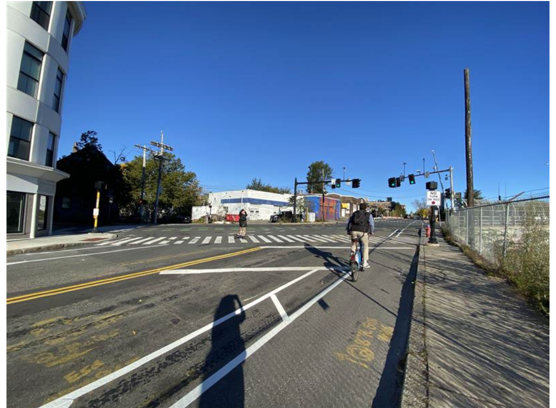
Above: New pavement markings for a protected bike lane on Webster Avenue.
