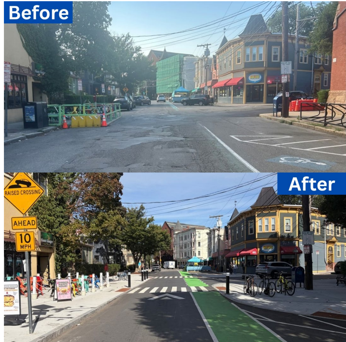
Completed raised intersection on Bow Street at Walnut Street.
