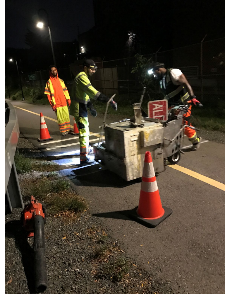
Above: City Contractors implementing new thermoplastic strips on the Community Path at Central Street.
